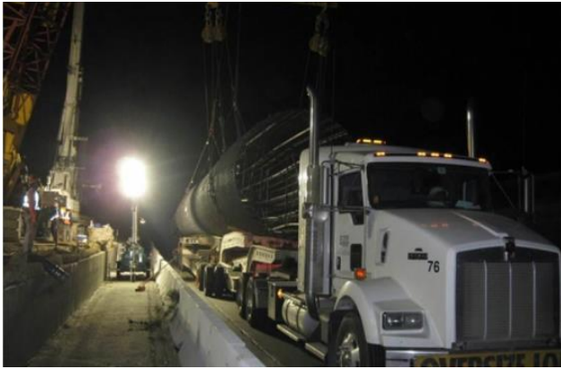
Figure 10: I-405 CIDH Rebar Cage Placement
