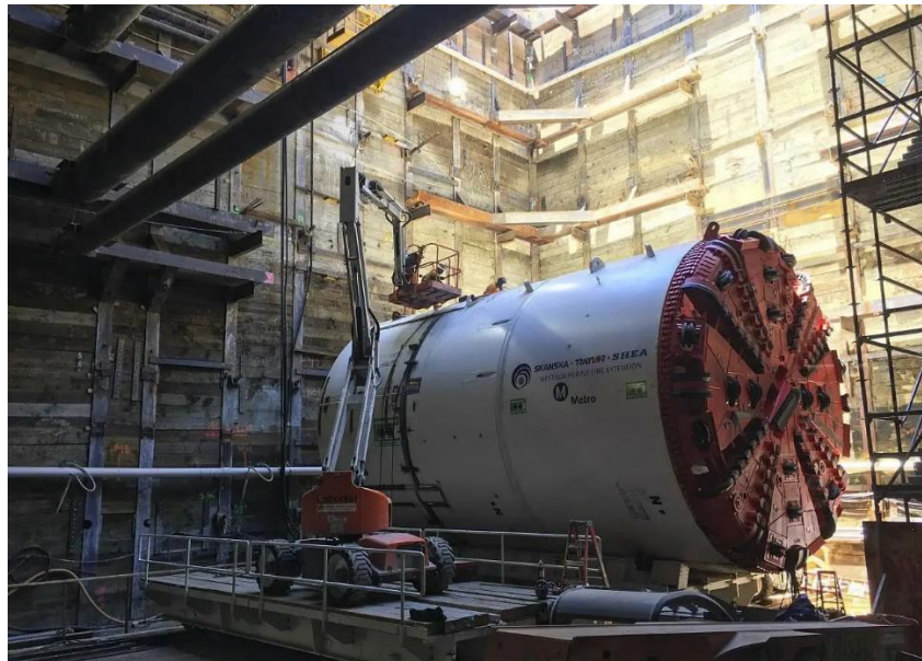
Figure 3-3. Tunnel Boring Machine
