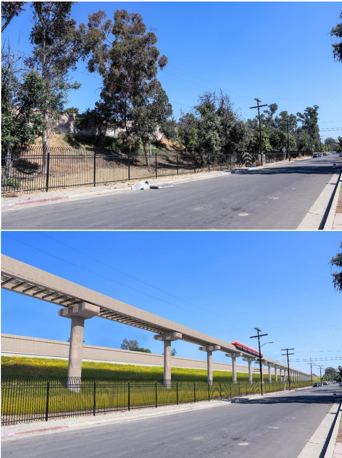
Figure 3.1-27. KOP 11 – Before and After Simulation View, View Looking West Toward the Aerial Alignment along I-405 and Firmament Avenue
