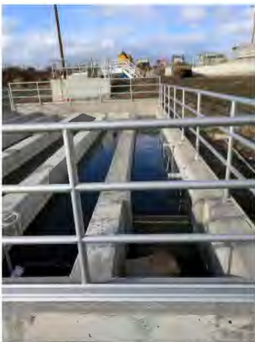
Figure 19. Chlorine contact chamber. Chlorine injection occurs in the upper structure in the background and dechlorination (sulfur dioxide injection) occurs at the chamber outfall in the foreground.
