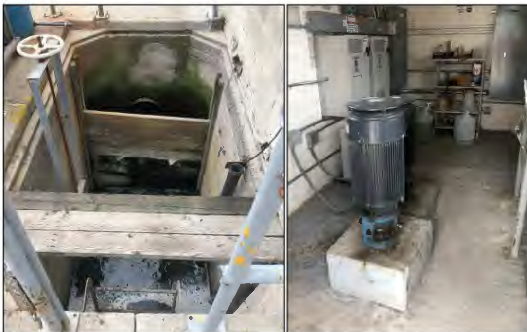
Figure 12. Recirculation flow control structure (left) and pump station to secondary clarifier (right).
