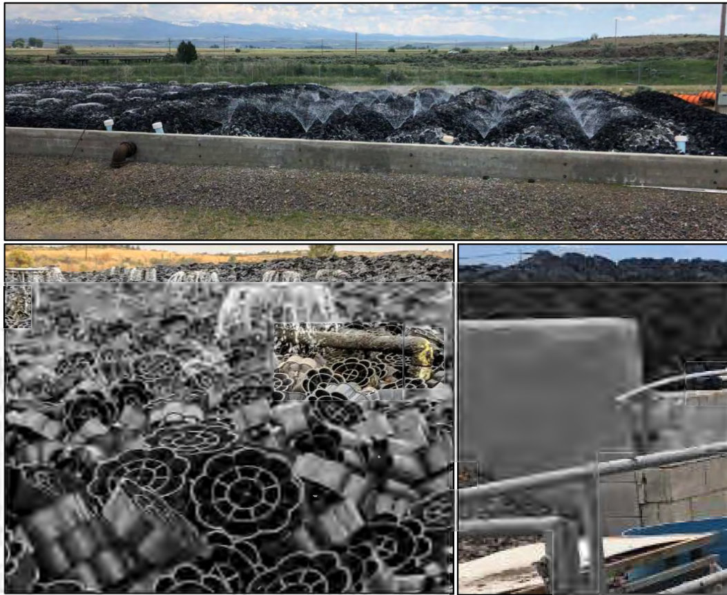
Figure 11. Trickling Filter (top) showing media (bottom left) and exterior wall where cracking has occurred in the CMU block wall (bottom right).
