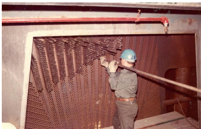
Figure 4: 1972 photo of installation of copper tubing for condenser for Unit 1. Source: PG&E.
