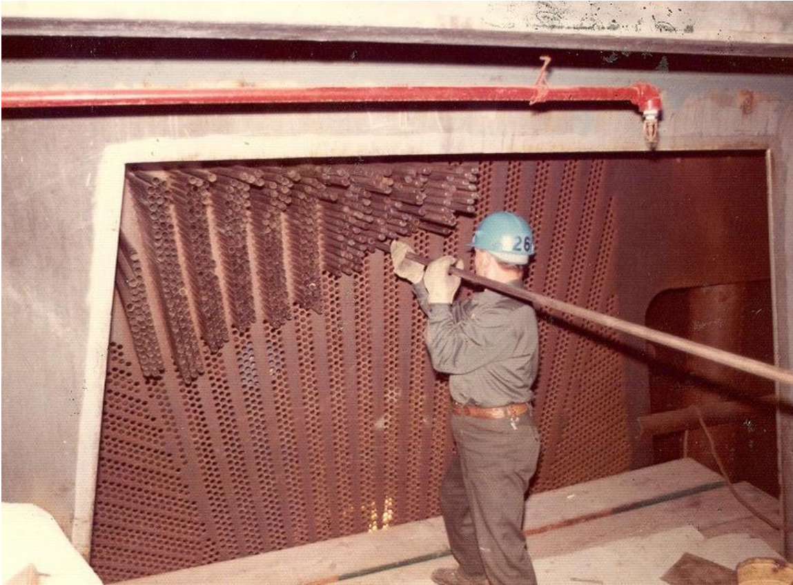
Figure 28. Undated photograph of the copper tubing in the Turbine Building that was replaced with titanium tubing to prevent toxins resulting from the chemical reaction between the copper and salt water.
