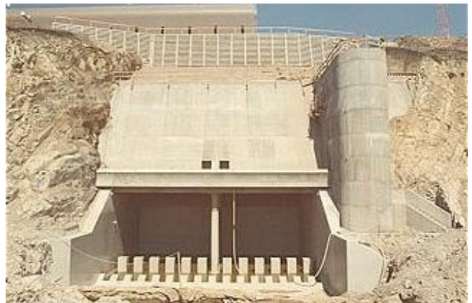
Figure 2: Undated photo of the Discharge Structure's outlet under construction, looking northeast at cove bed with the north half of the Turbine Building visible above. The outlet is currently submerged. Source: PG&E.
