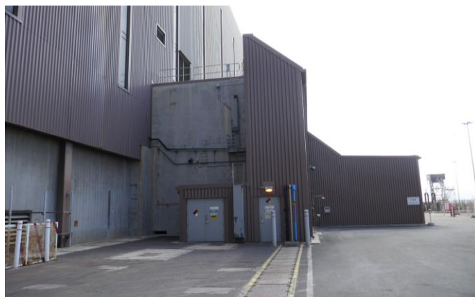
Figure 5: One of two one-story additions at the west façade of the Turbine Building enclosing the structural buttress reinforcements and additional equipment, looking south. Source: Page and Turnbull, 2021.
