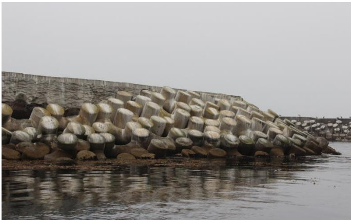
Figure 1: East Breakwater from Intake Cove, with visible concrete tribars, looking west.
