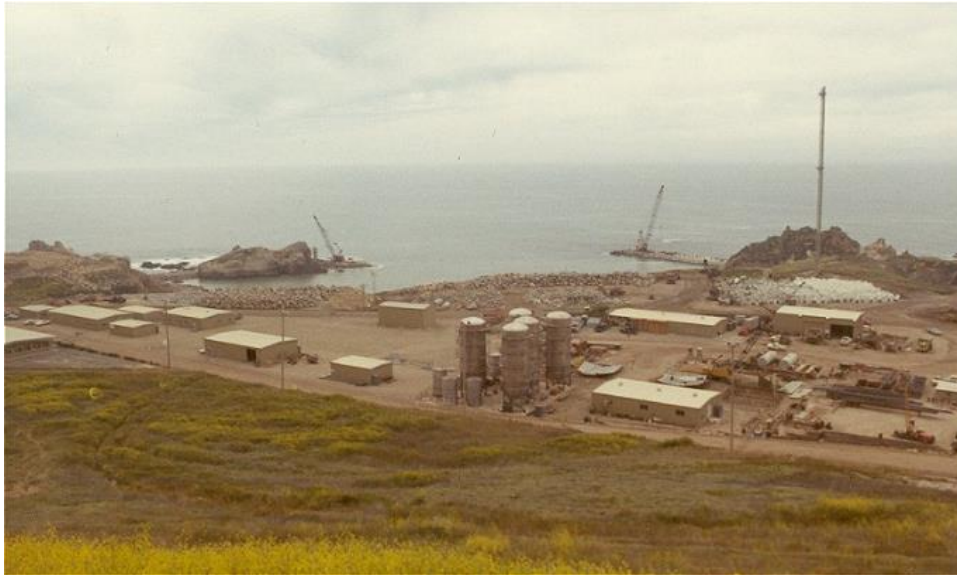
Figure 22. Support buildings and structures in the fabrication yard in April 1971 (currently Parking Lot 6 in Zone 5). In the background, the breakwaters are under construction in the intake cove. Source: Pacific Gas and Electric Company.
