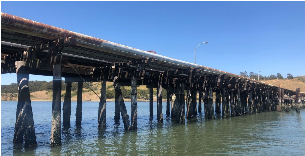
Figure 2-3. The Causeway (Oriented East-West) of the Point Orient Wharf, Primarily Supported on Jacketed/Wrapped Wooden Piles
