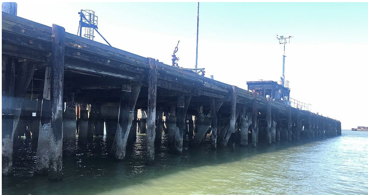
Figure 2-5. Concrete and Steel Fendering Protecting the Main Wharf
