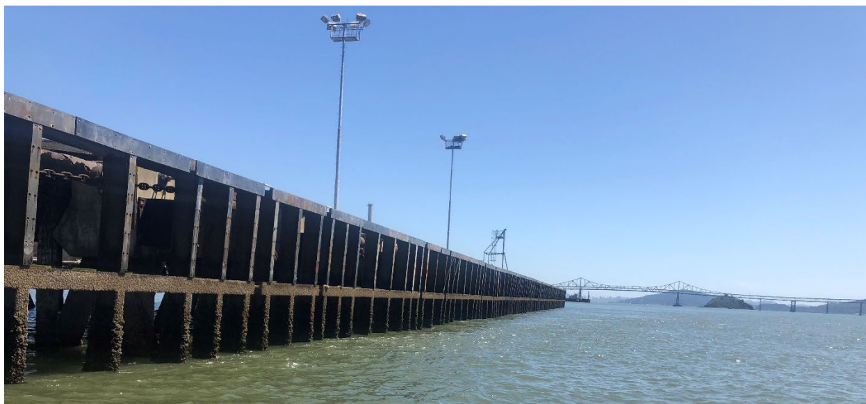
Figure 2-5. Concrete and Steel Fendering Protecting the Main Wharf
