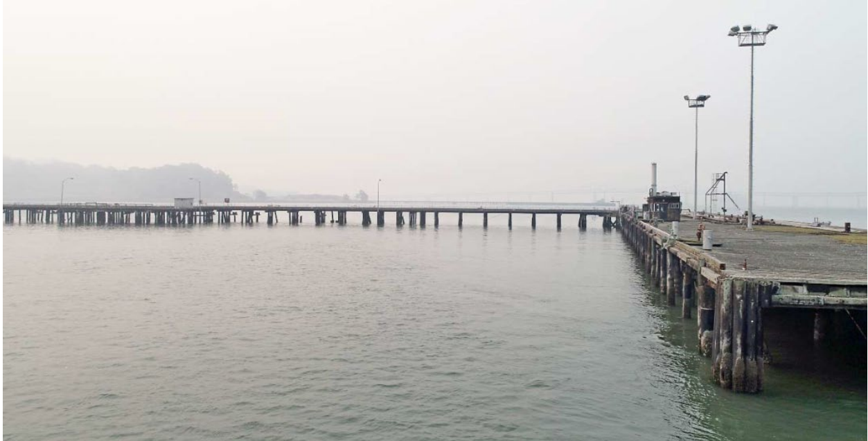
Figure 2-3. The Causeway (Oriented East-West) of the Point Orient Wharf, Primarily Supported on Jacketed/Wrapped Wooden Piles
