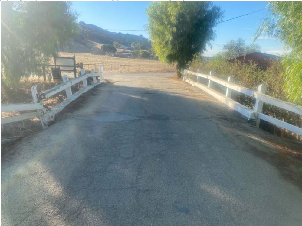
Photo 6. View of the bridge looking west toward Foxen Canyon Road.
