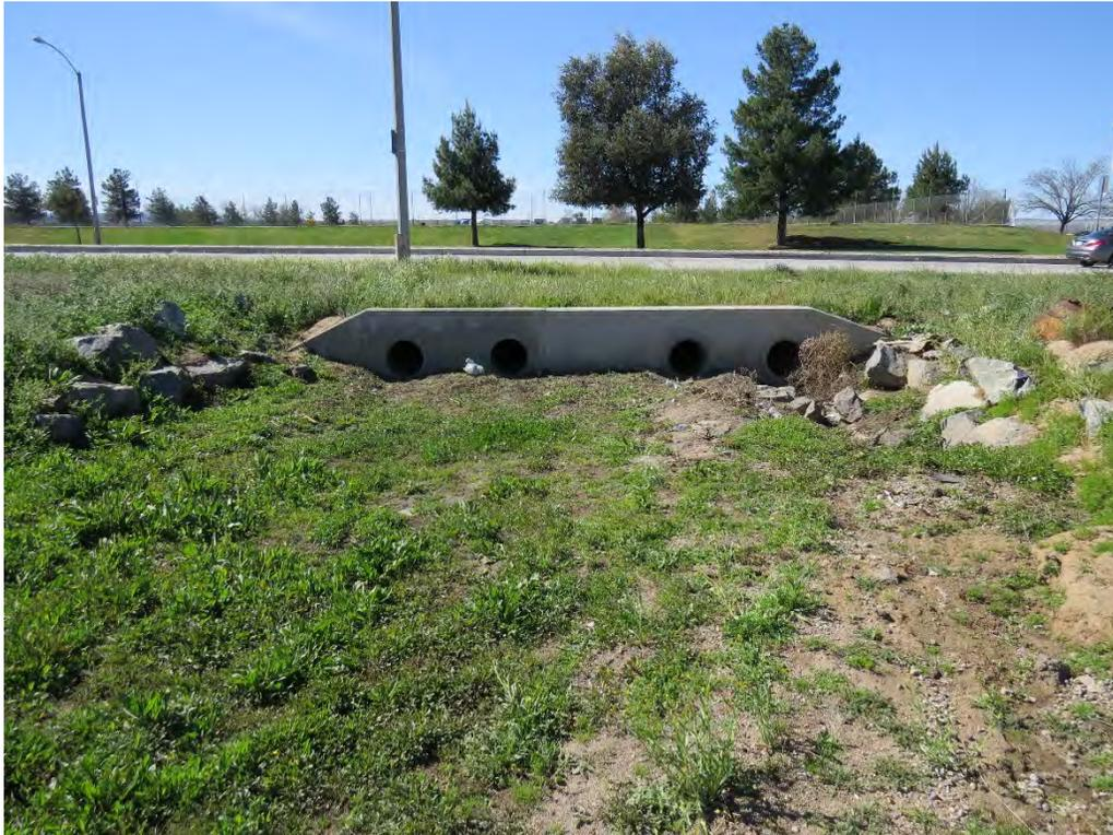
**Photograph 20:** Looking at the western terminus of the swale where it extends under Indian Avenue, via four 24-inch culverts, and connects with a water detention basin on the southwest corner of the intersection of Ramona Expressway and Indian Avenue.
