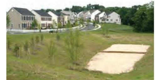
Sand filter at the base of the bioswale promotes infiltration.
