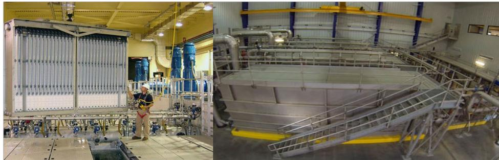
**Image 2-11a MBR Filtration Module at the WWTP**
