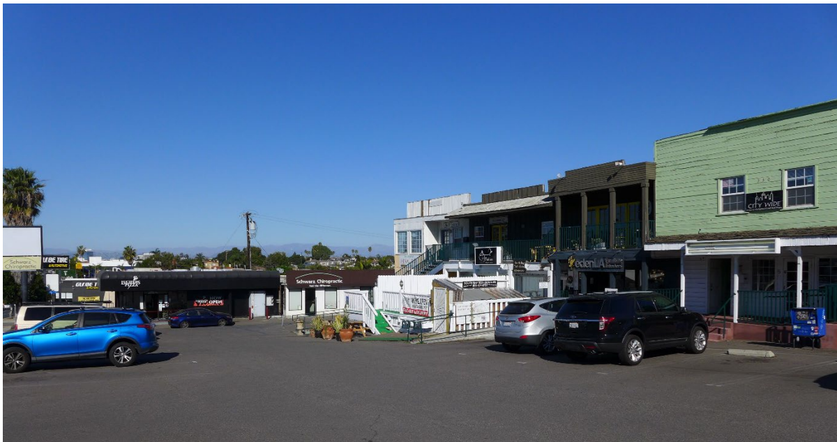
Photograph 2. View of Lucifers Pizza and parking lot looking north from east side of Sepulveda Boulevard
