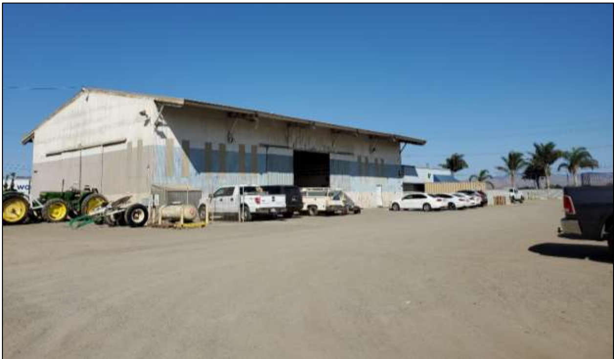
Photograph 2. Existing warehouse building on north portion of project site facing southeast (September 29, 2020).
