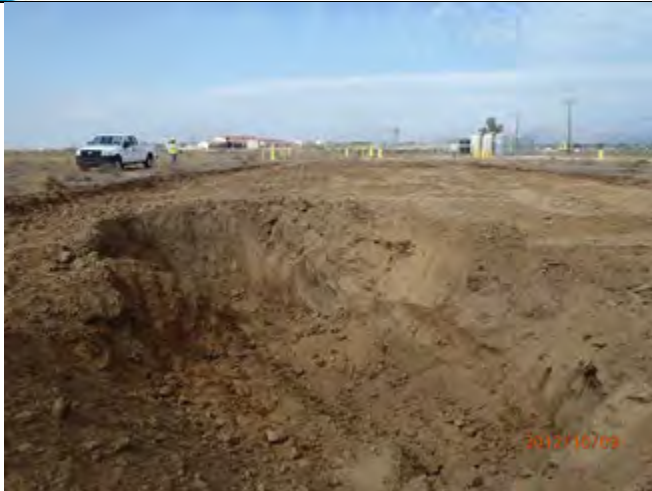
Hot spot area excavated out to brown soil, gray soil max depth observed was 6 feet
