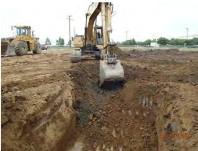
Excavating and removing gray soils down to brown soil with very low odor levels.
