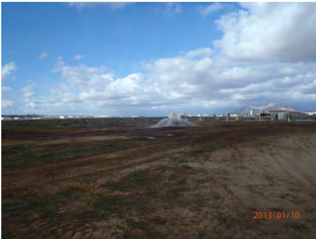
Wet site down to create a dirt crust to help prevent dust and to enhance grass growth
