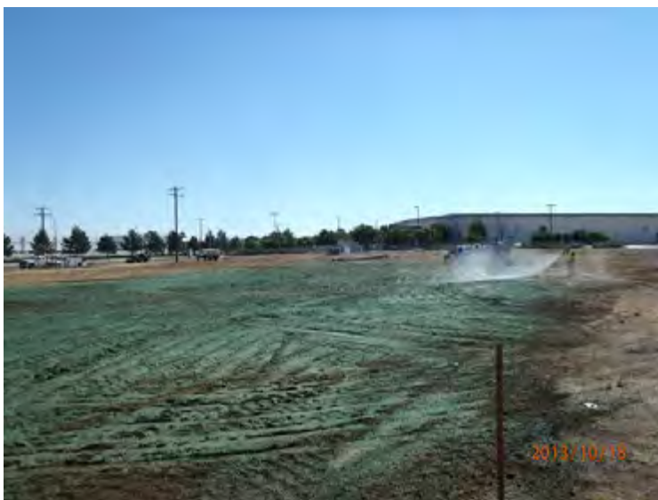
Hydro Seeding the excavation area, looking S from NW Corner
