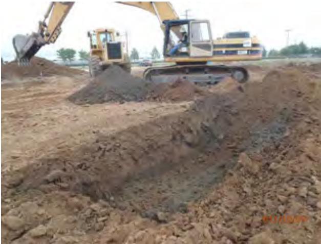
Located hot spot of grayish soil with low PID reading average around 15 to 20 ppm
