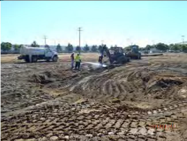
Soil conditioning and compacting excavation with Norcal performing soil compaction testing, Looking South
