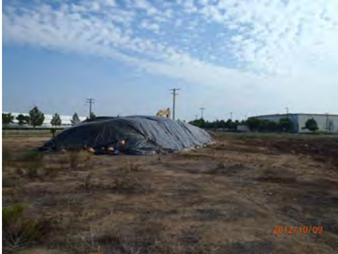
Stock pile approx. 8x25x70 feet = 518 cu yards, covered and secured awaiting analytical results
