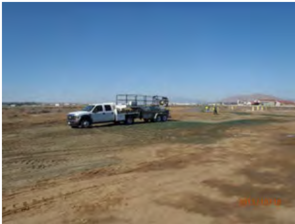
Hydro Seeding the excavation area, looking NW
