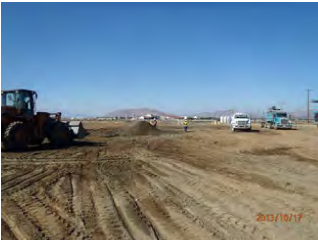
Soil conditioning and compacting excavation with Norcal performing soil compaction testing, Looking North
