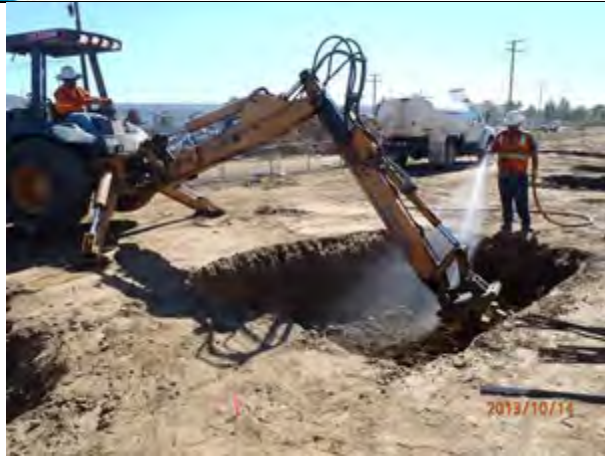
Soil conditioning and compacting excavation
