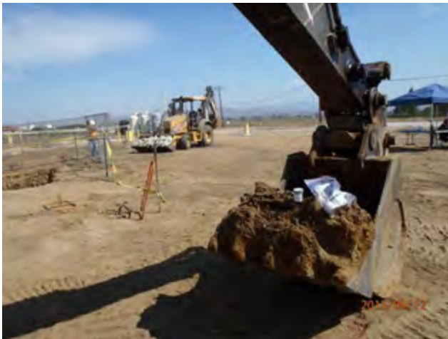
Obtaining confirmation samples and installing security fencing
