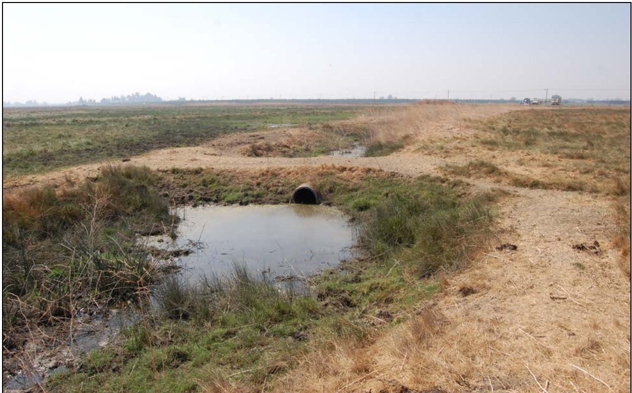
Figure 10: 78-Acre Parcel – view southwest towards Canal School Road along drainage that extends diagonally through the parcel
