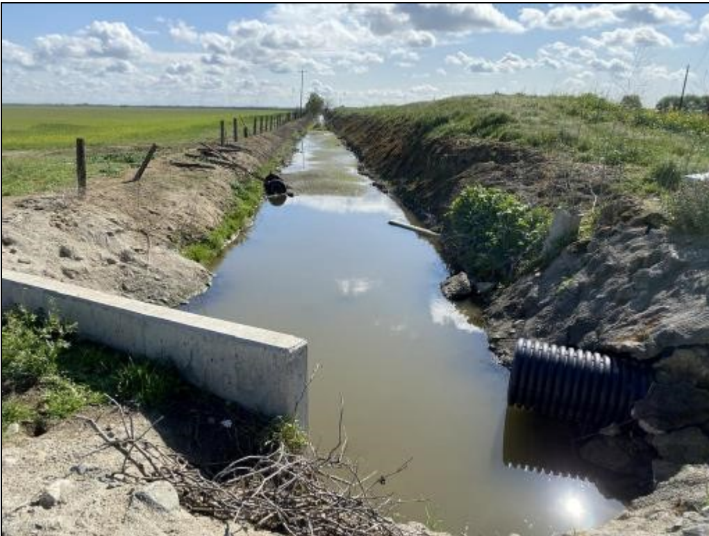
View east along Miller Ditch from near East Inyo Rd (Vollmar Natural Lands Consulting)
