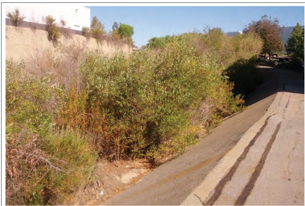
July 23, 2014. View upstream showing overview of Reach 110 north of bridge.
