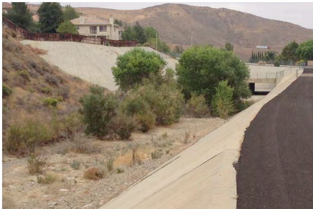
July 15, 2014. View downstream showing terminus of Reach 102.
