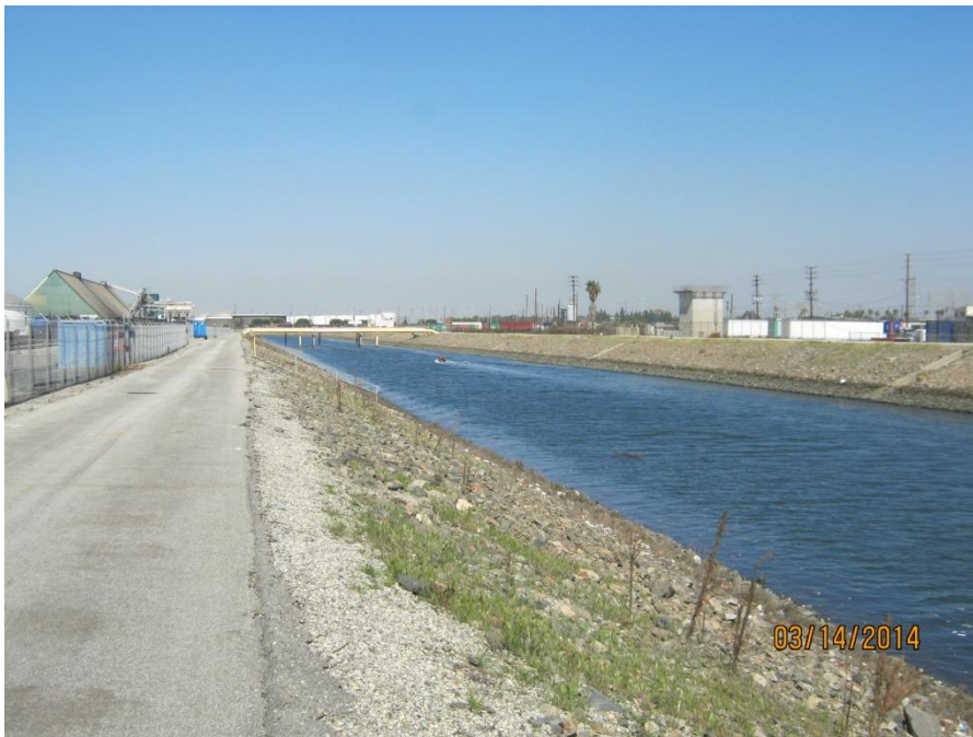
Photo 7. Photo showing Dominguez SBC between Alameda Street and Sepulveda Blvd. This portion of the channel is sparsely vegetated and is bordered by an oil refinery. Photo facing northwest.
