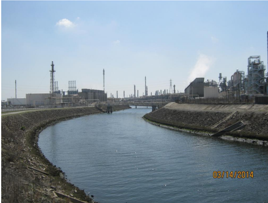
Photo 7. Dominguez SBC between 223 rd Street and Alameda Street. The channel flows through a power plant and is sparsely vegetated along the banks. Photo facing southeast.
