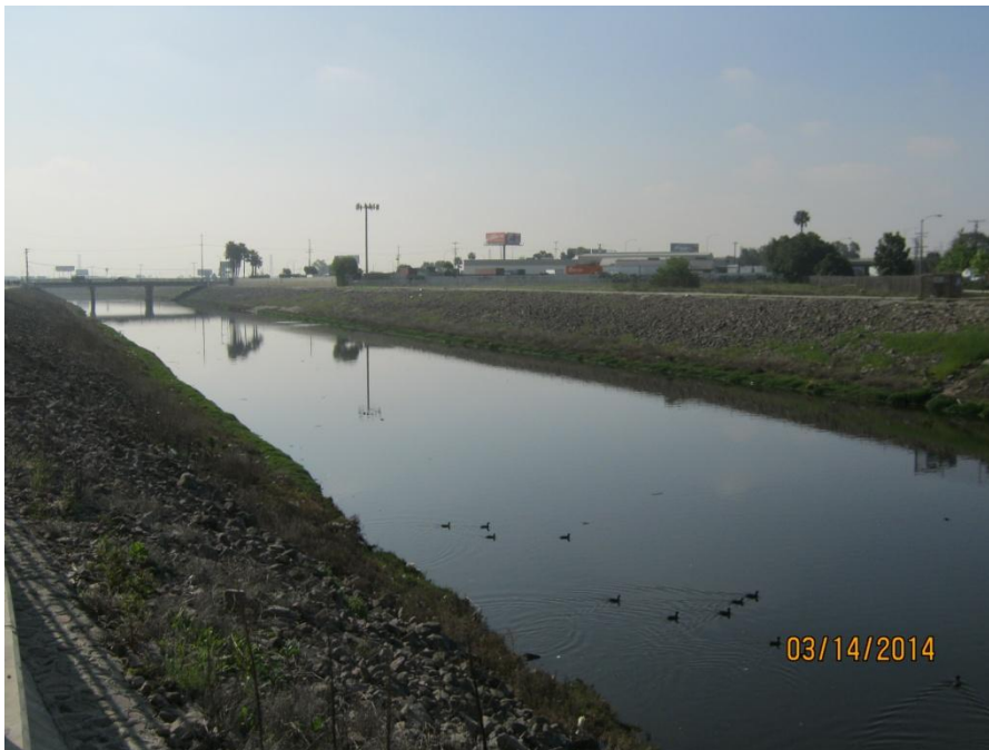
Photo 4. Dominguez SBC between S. Main Street and Del Amo Blvd. Banks are moderately vegetated. This portion of the channel is bordered by open space. Photo facing southeast.
