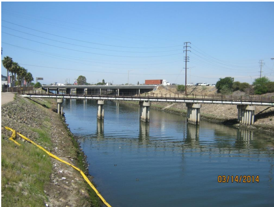
Photo 6. Photo showing the channel between Carson Street and 223 rd Street. Banks along the west side of the channel are more evenly vegetated. The bridges located throughout the channel could provide potential nesting habitat for birds. Photo facing northwest.
