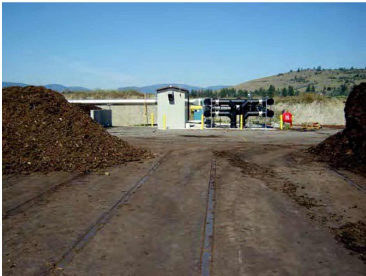
Figure 2: Aeration floor compost system (with spargers)
