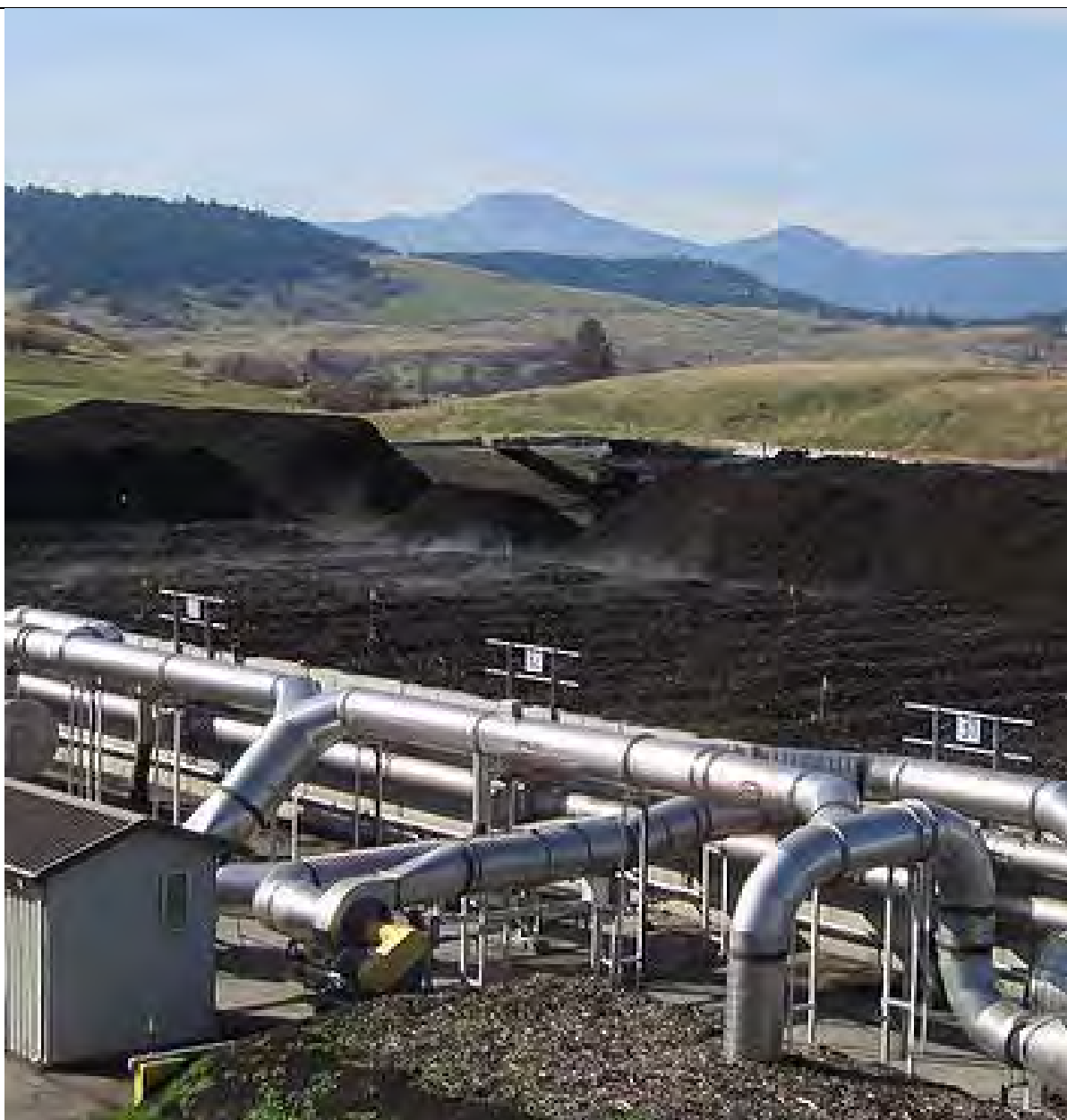
Figure 3: Aerated Static Pile with Fan Group and Ducting
