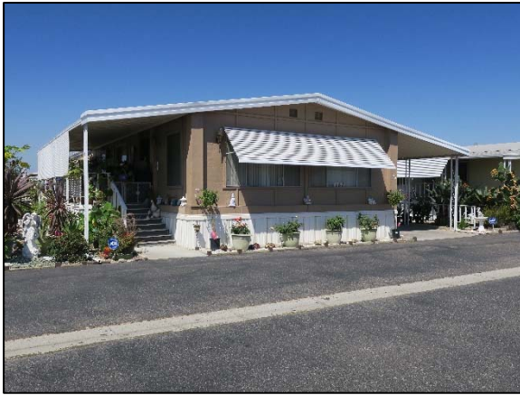
Example of typical older unit.
