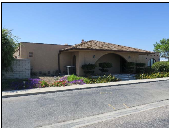
Community building east façade, view northwest.
