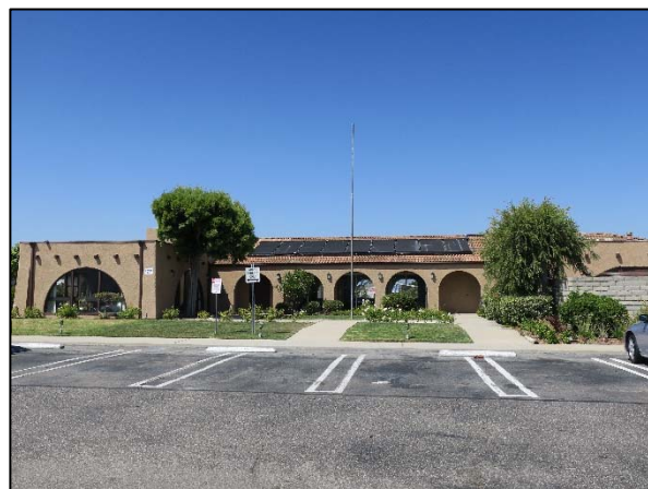
Community building south façade, view north.
