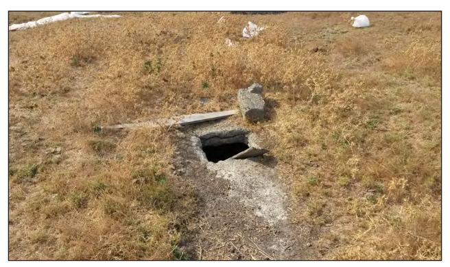
**Photo 5:** A possible septic vault near the building foundation remnants.
