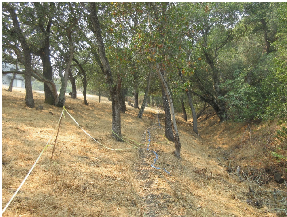
Photo 2: View of proposed pathway alignment and existing informal footpath. An existing residence can be seen in the upper left corner of the photo.
