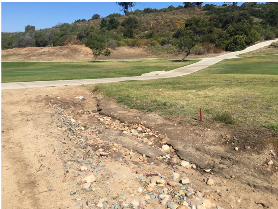
Photo 6. View of project study area on Balboa Park Golf Course and small streambed facing northwest. June 27, 2017.
