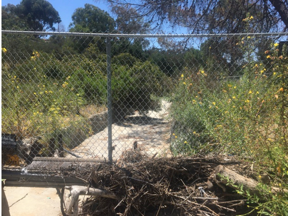
Photo 7. View of concrete channel south of 28 th Street and Maple Street, which passes through a private residence, facing south. June 27, 2017.
