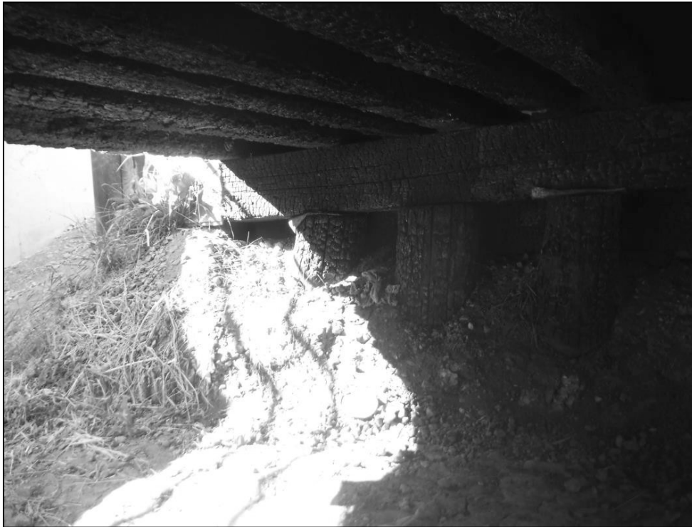
Photo 1: Abutment 1 – Typical fire damage and leaking ballast.
