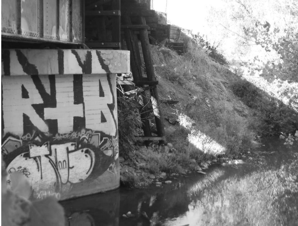
Photo 4: Failing channel protection on northeast embankment.
