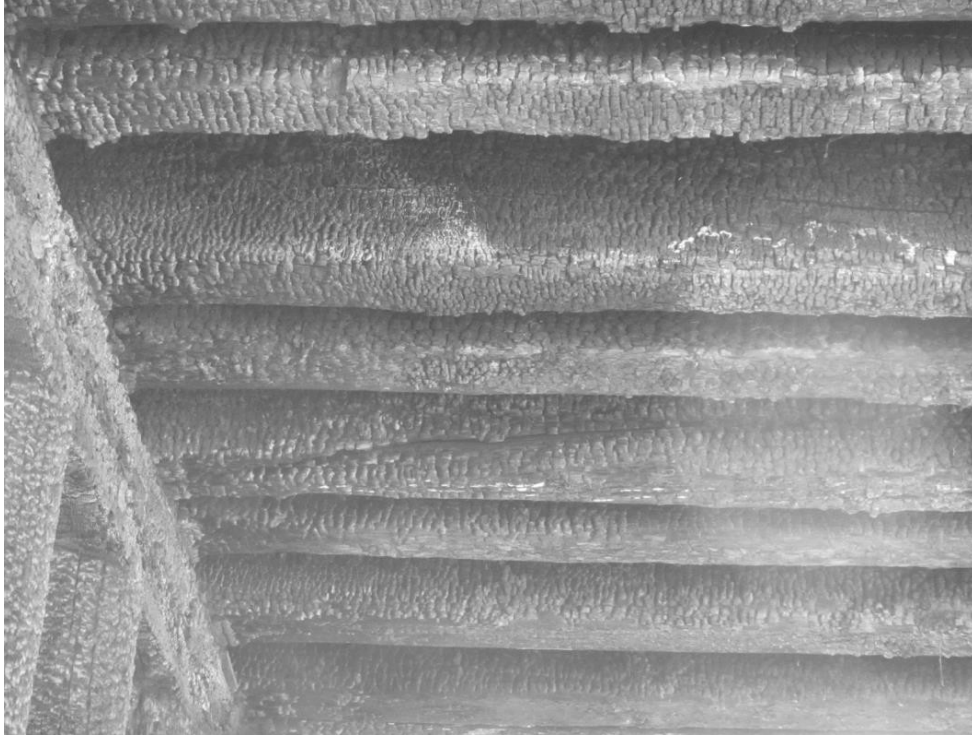
Photo 2: Typical stringer span fire damage.
