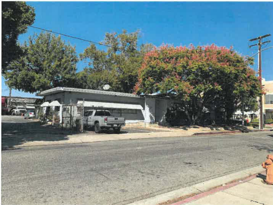
Photo 4: View from Boyle Avenue facing into the project site. 573 Bickett St., Huntington Park, CA 1 Story 2 Industrial.
