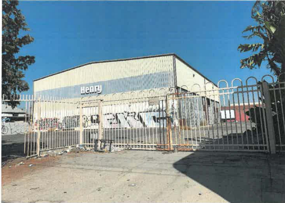
Photo 3: View from Slauson Avenue facing into the project site. 2601 Slauson Ave., Huntington Park, CA 1 Story – Industrial.
