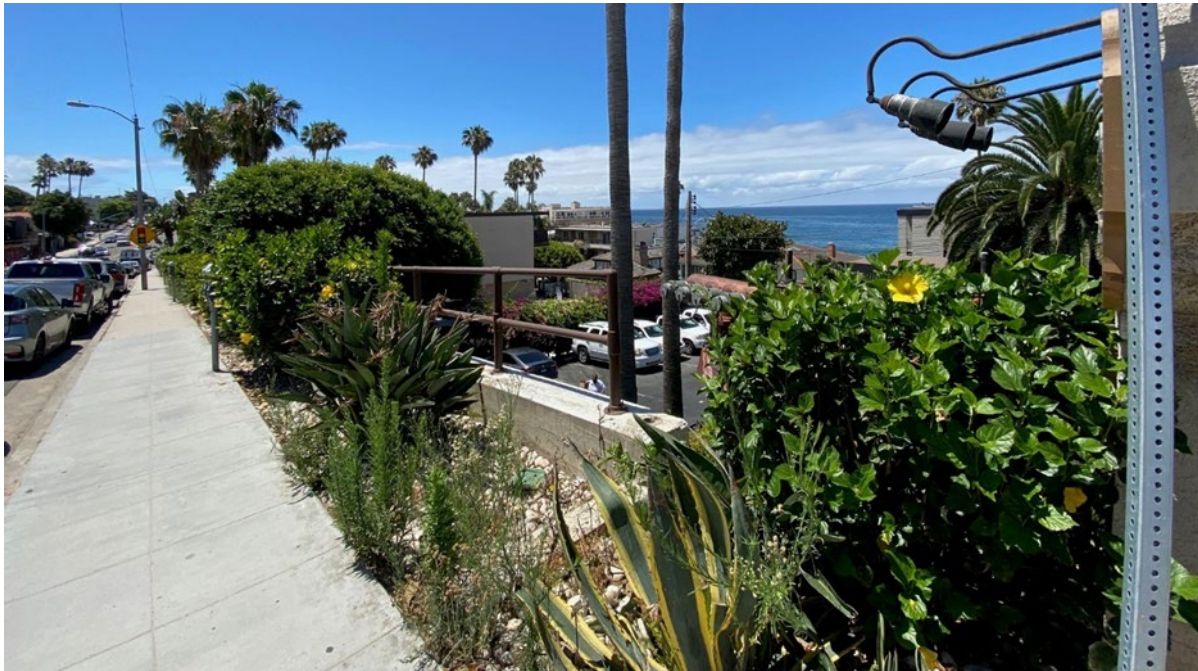
Figure 7d: View of existing Pacific Edge Hotel from the sidewalk at the intersection of SR-1 and Sleepy Hollow Lane.
