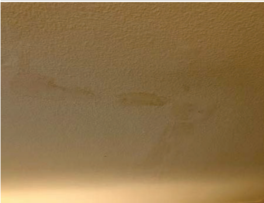
24. Marina Inn, Room 129 – View of water staining/damage on bedroom ceiling.
