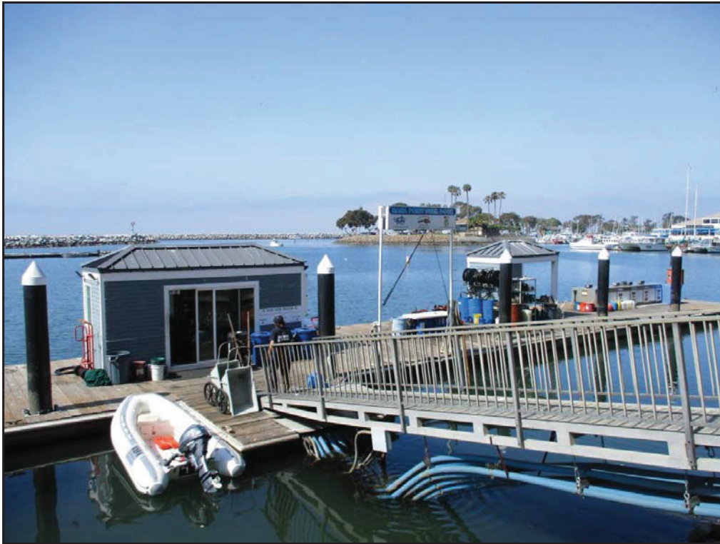
5 : Dana Point Fueling Dock, facing south. Fuel-bearing piping (blue) was observable beneath the dock.
