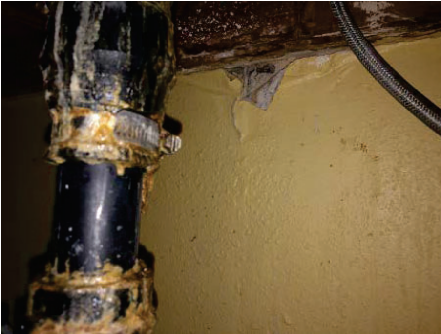
25. Marina Inn, Laguna Niguel Room - View of water staining/damage and suspect microbial growth underneath the sink.
