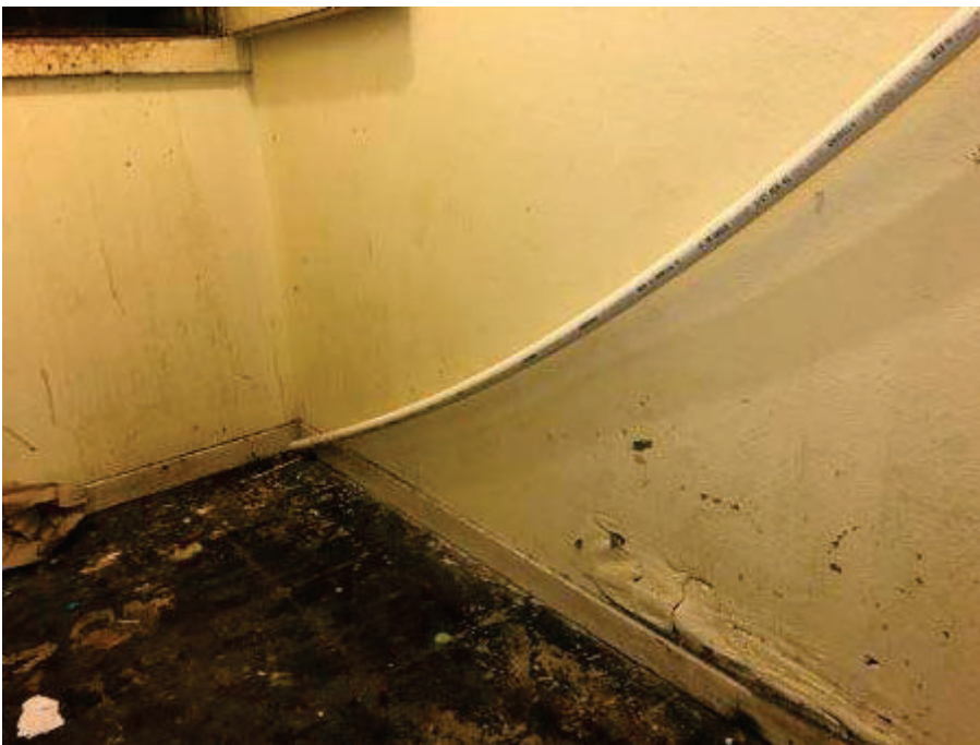
29. Marina Inn, Room T3 – View of water staining/damage on North and East walls.
