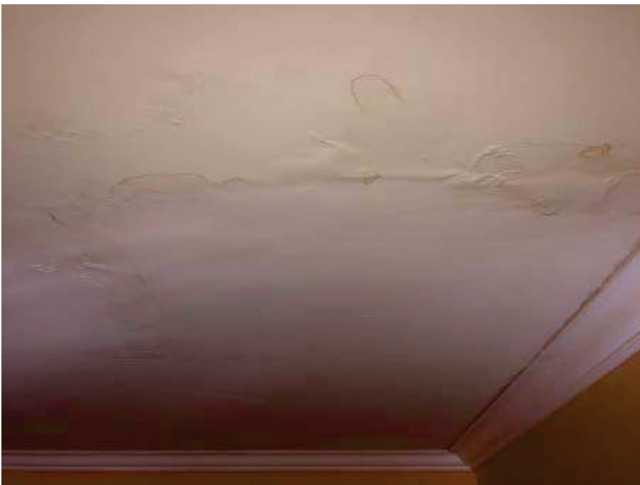
35. Marina Inn, Room 330 – View of water staining/damage on bedroom ceiling.
