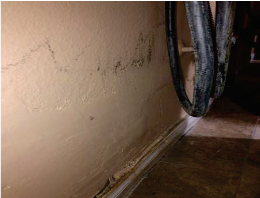
28. Marina Inn, Guest Laundry Room – View of water staining/damage and some suspect microbial growth behind the fourth laundry machine on East wall
