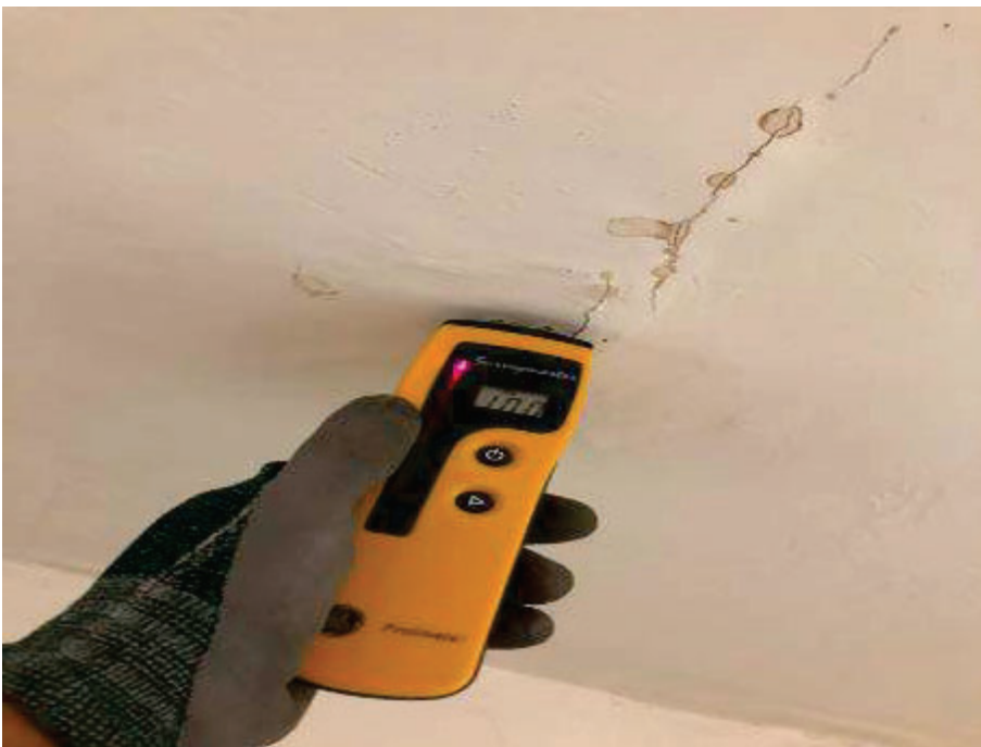
55. Marina Inn, Dana Point Room – View of elevated moisture readings on ceiling.
