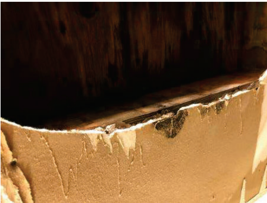
33. Marina Inn, Room 3D – View of suspect microbial growth on the drywall ceiling
