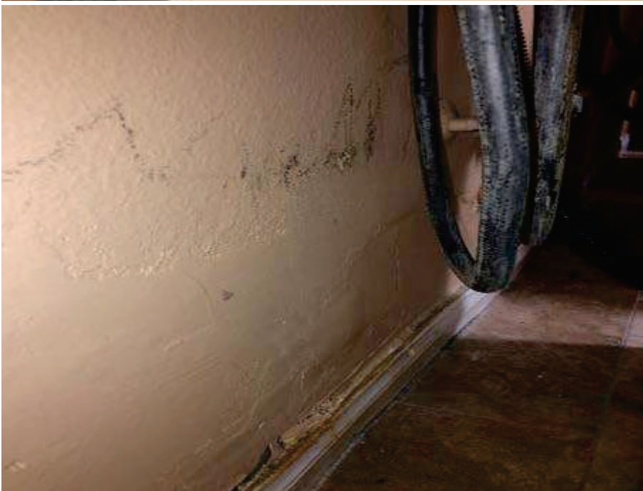
56. Marina Inn, Guest Laundry Room – View of water staining/damage and some suspect microbial growth behind the fourth laundry machine on East wall
