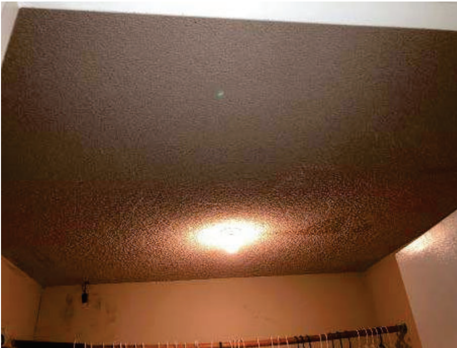
28. Marina Inn, Room L3 – View of three different water stains on ceiling.
