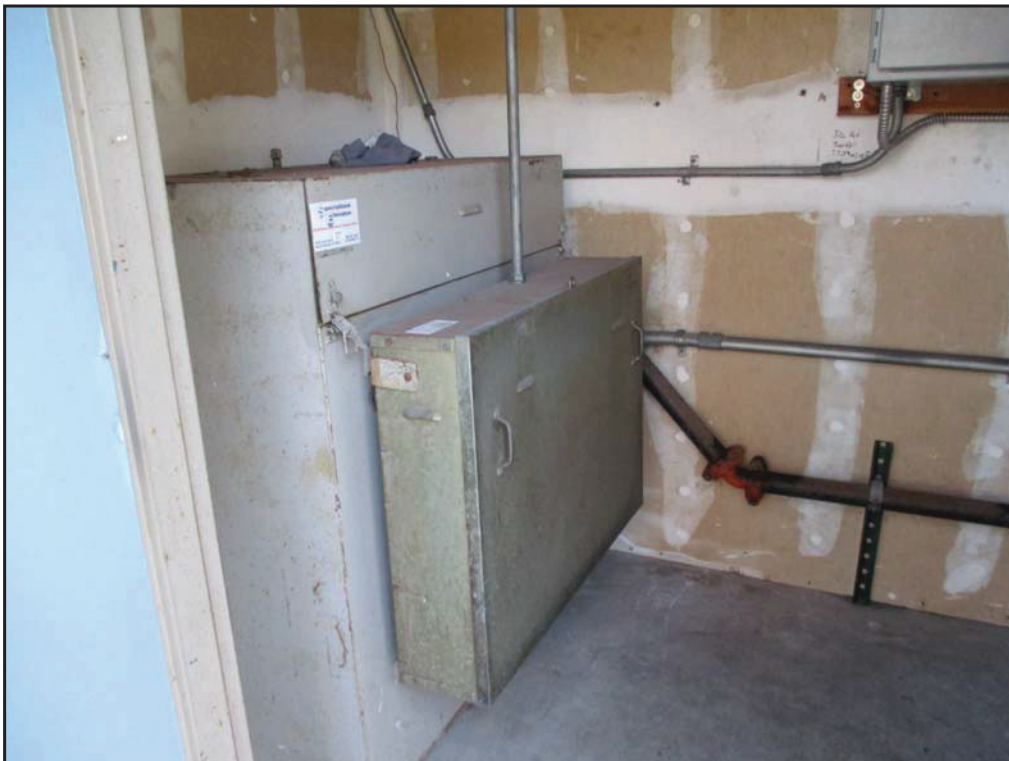
66 : East Basin Building 4 - The Marina at Dana Point building (34555 Casitas Place) - hydraulic elevator AST closet
