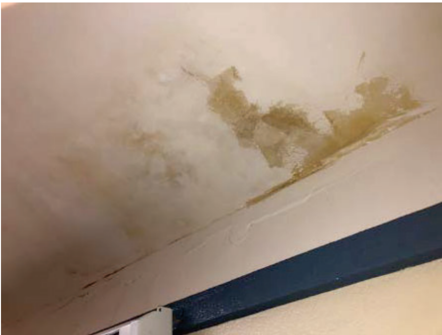
26. Marina Inn, Dana Point Room – View of water staining/damage on ceiling.
