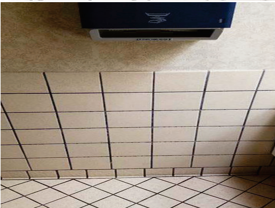
22. Building 4 – View of lead-based ceramic wall tile in the 2 nd Floor Women's Restroom.
