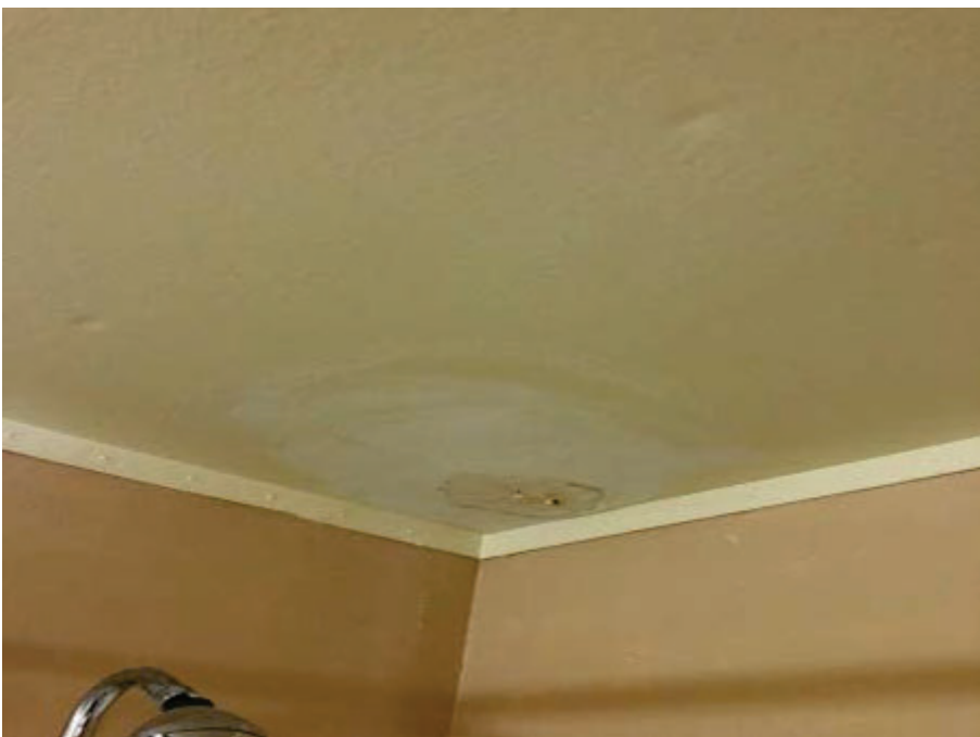
32. Marina Inn, Room 100 (Boardroom) – View of water staining/damage on bathroom ceiling above shower.
