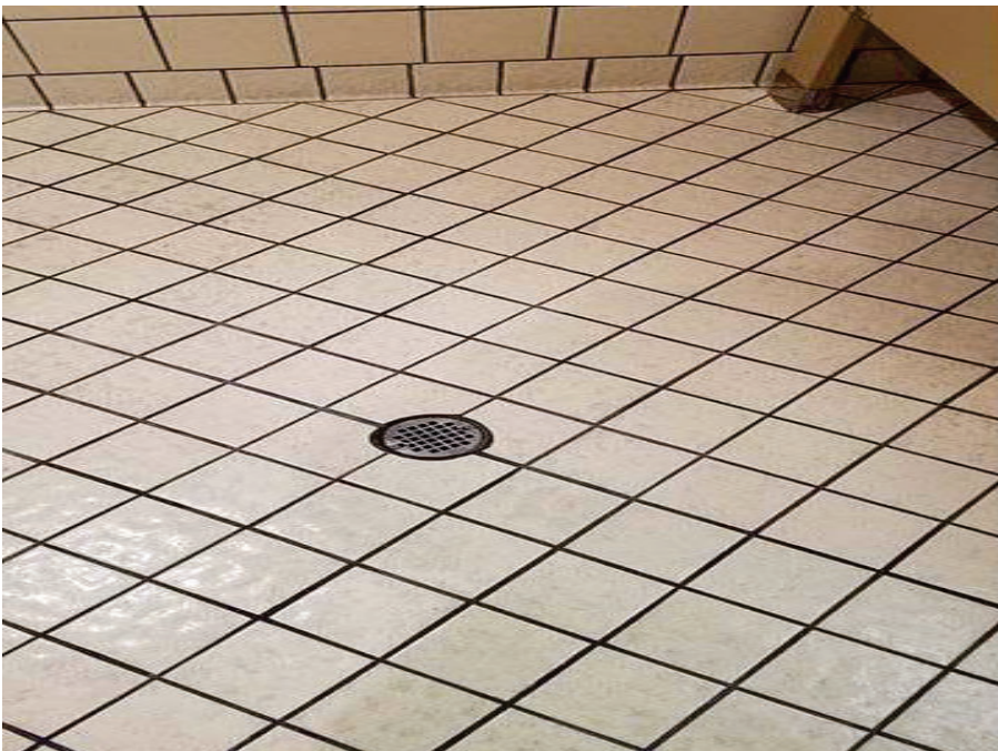
18. Building 4 – View of lead-based ceramic floor tile in the 2 nd floor Men's Restroom.
