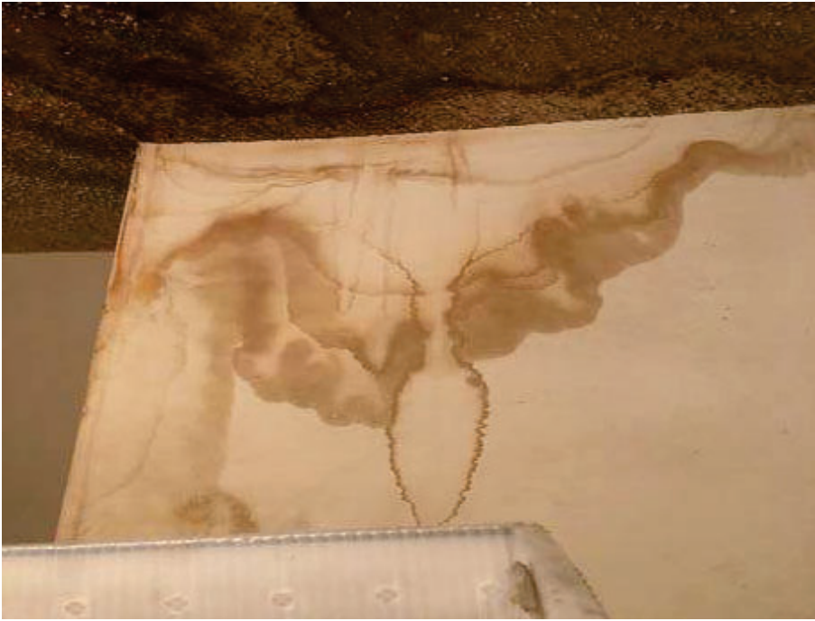
45. Marina Inn, Room 3A – View of water staining/damage on West wall.
