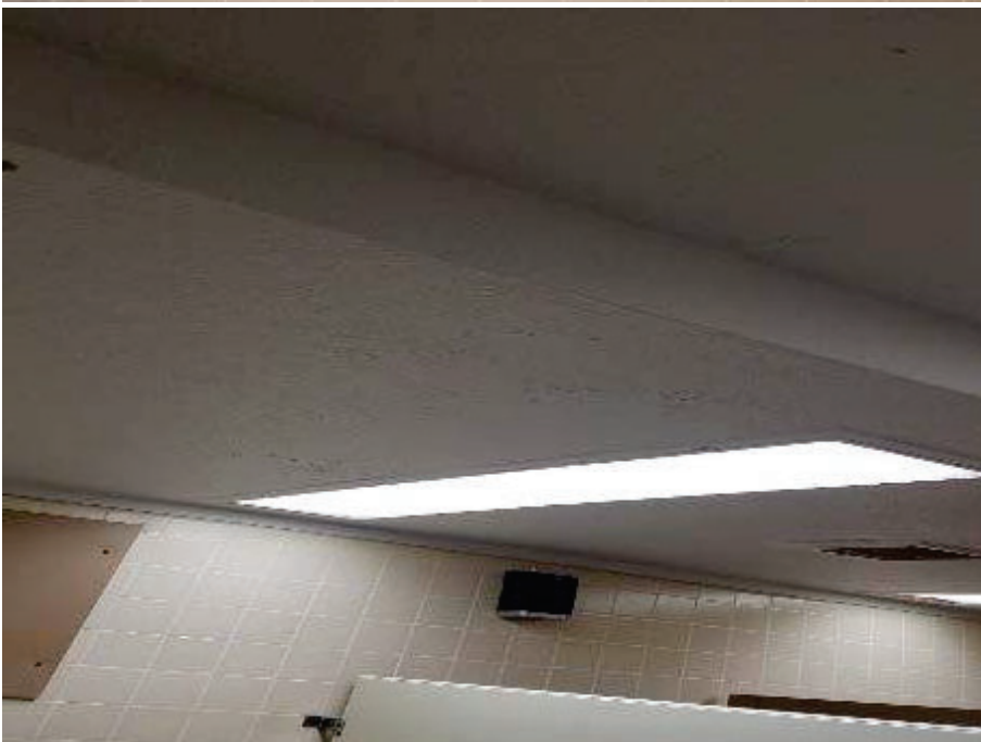
16. Building 3 – View of lead-based plaster wall in the 1 st Floor Women's Restroom ceiling.
