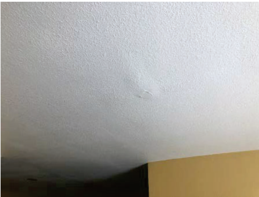
25. Marina Inn, Room 361, View of water damage at bedroom ceiling.
