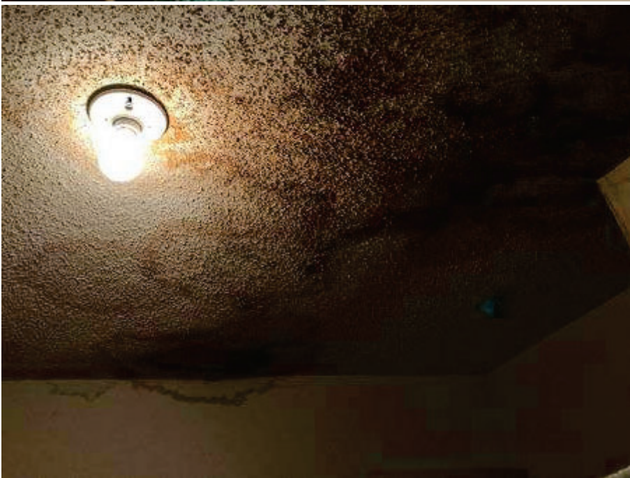
44. Marina Inn, Room 3A – View of water staining and suspect microbial growth across ASO ceiling.
