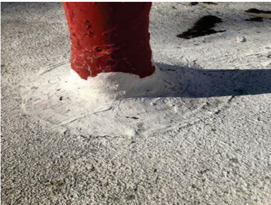
9. Marina Inn – View of ACBM gray penetration mastic.
