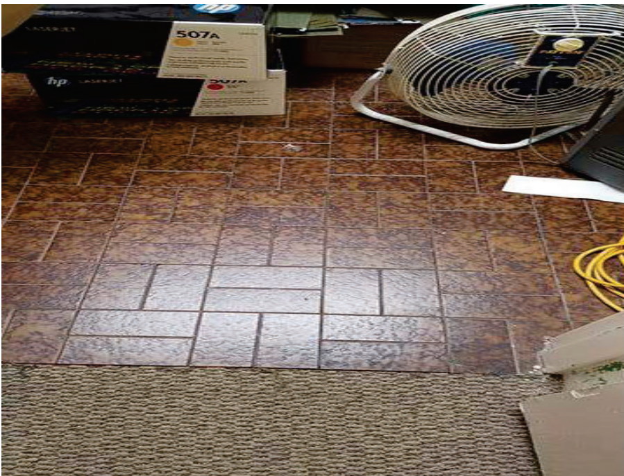
23. Building 4 – View of lead-based ceramic floor tile in the 2 nd Floor Storage Room.
