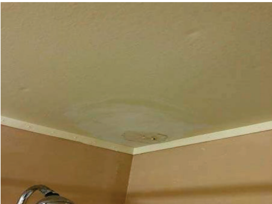
60. Marina Inn, Room 100 (Boardroom) – View of water staining/damage on bathroom ceiling above shower.
