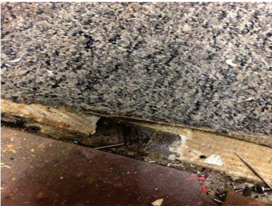
13. Building 3 – View of ACBM 12"x12" tan floor tile with mastic underneath carpet.
