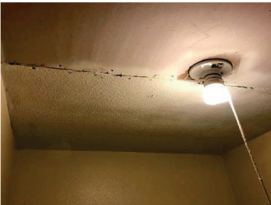
30. Marina Inn, Room T3 – View of drywall ceiling where it has been previously removed and patched.
