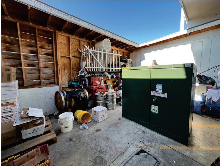
25. Pad-mounted electrical transformer
