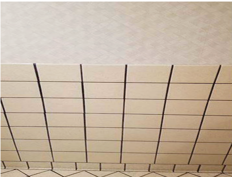
19. Building 4 – View of lead-based ceramic wall tile in the 2 nd Floor Men's Restroom.
