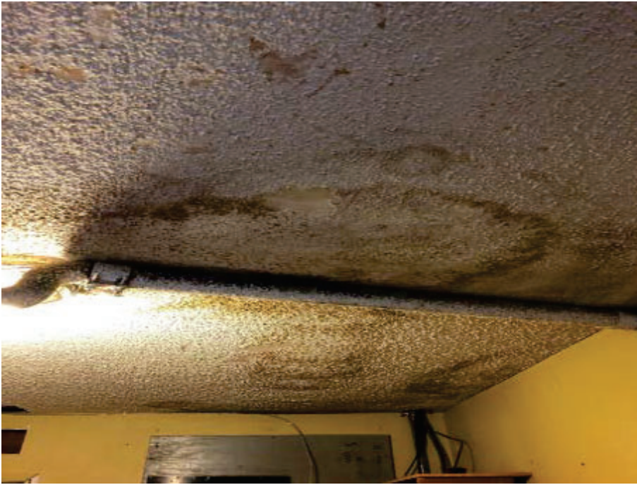
21. Marina Inn, Room 2C – View of water staining/damage on ASO ceiling.
