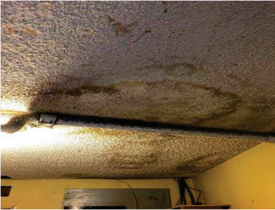
49. Marina Inn, Room 2C – View of water staining/damage on ASO ceiling.
