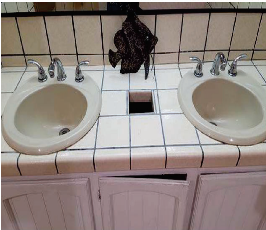
20. Building 4 – View of lead-based ceramic countertop tile in the 2 nd Floor Men's and Women's Restroom.
