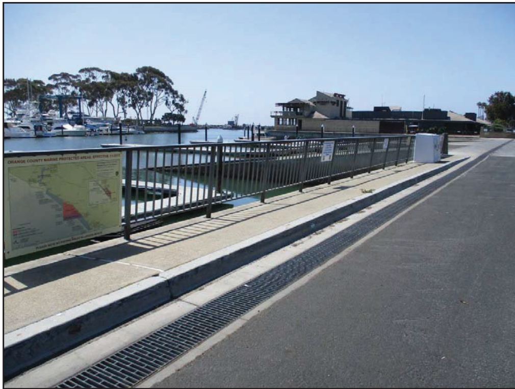
19 : Embarcadero at Dana Point boat wash trench drain
