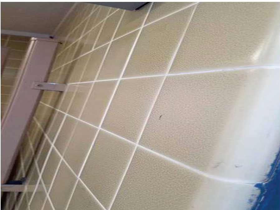
17. Building 3 – View of lead-based ceramic wall tile in the 1 st Floor Women's Restroom.
