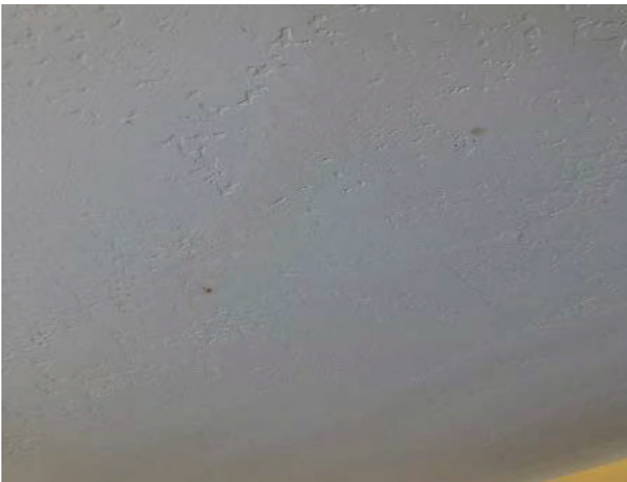
51. Marina Inn, Room 128 – View of water staining spots on bedroom ceiling.
