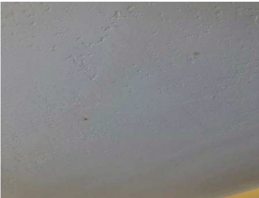
23. Marina Inn, Room 128 – View of water staining spots on bedroom ceiling.
