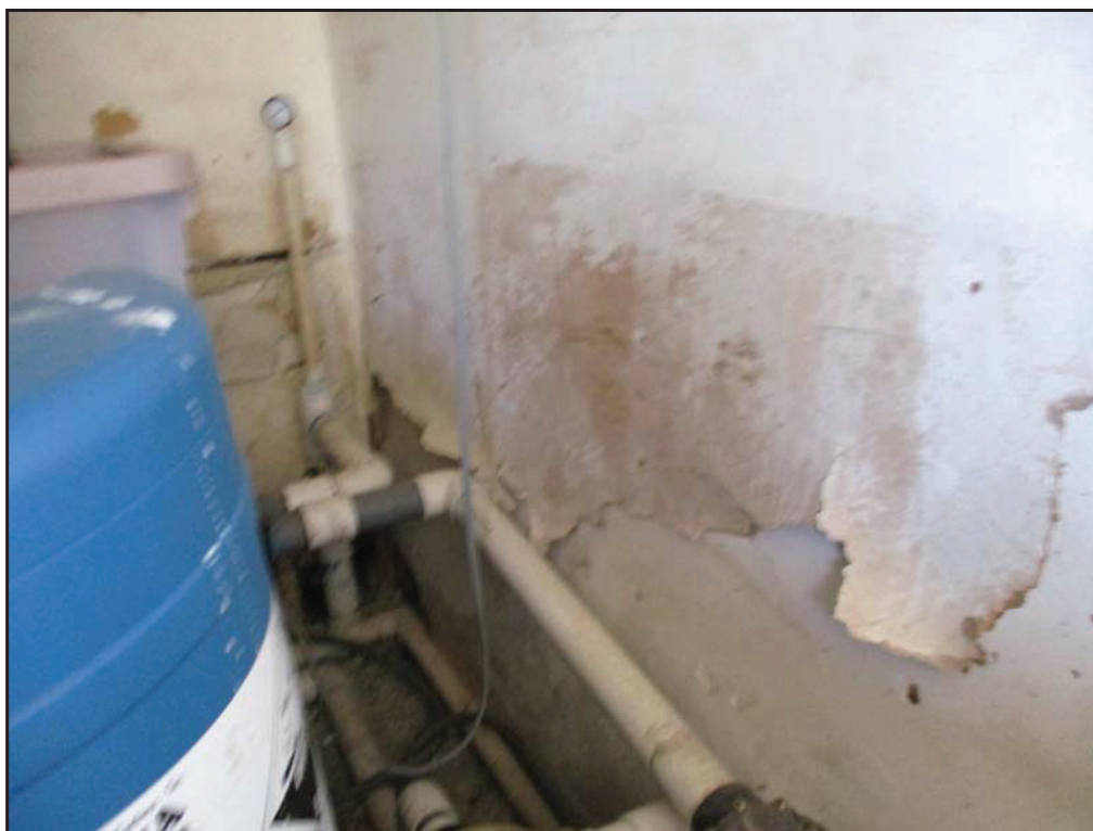
27 : Dana Point Marina Inn - damage to wall surface in pool equipment & boiler room
