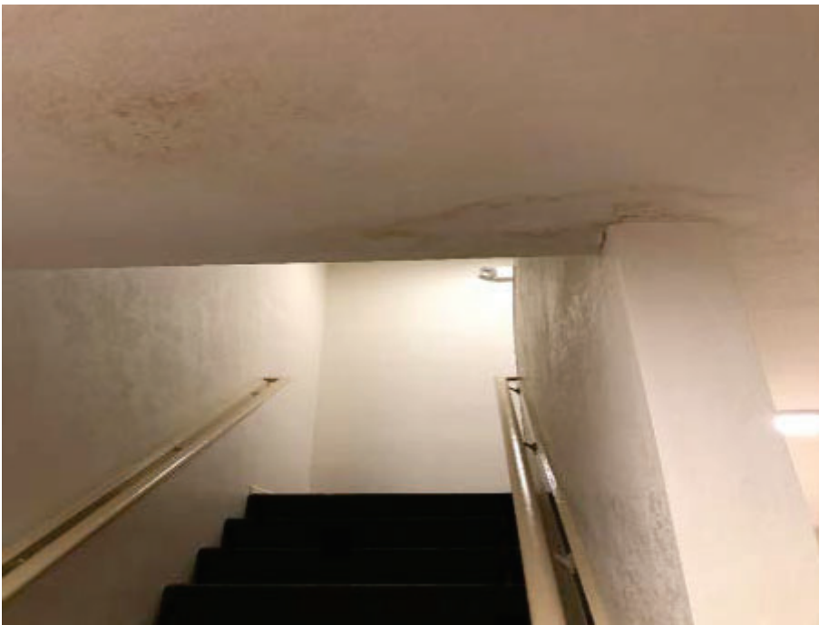
22. Marina Inn, 2nd Floor South Stair Landing – View of water staining/damage on ceiling.
