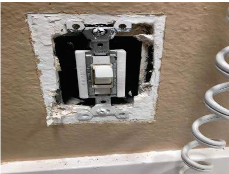
2. Marina Inn – View of the ACBM drywall joint compound.
