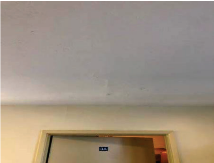
46. Marina Inn, Elevator landing adjacent to room 3A - View of water damage on drywall ceiling.
