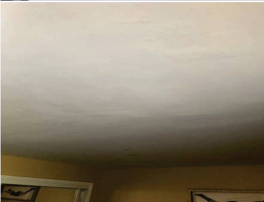
12. Marina Inn, Room 321 – View of water damage on bedroom ceiling.
