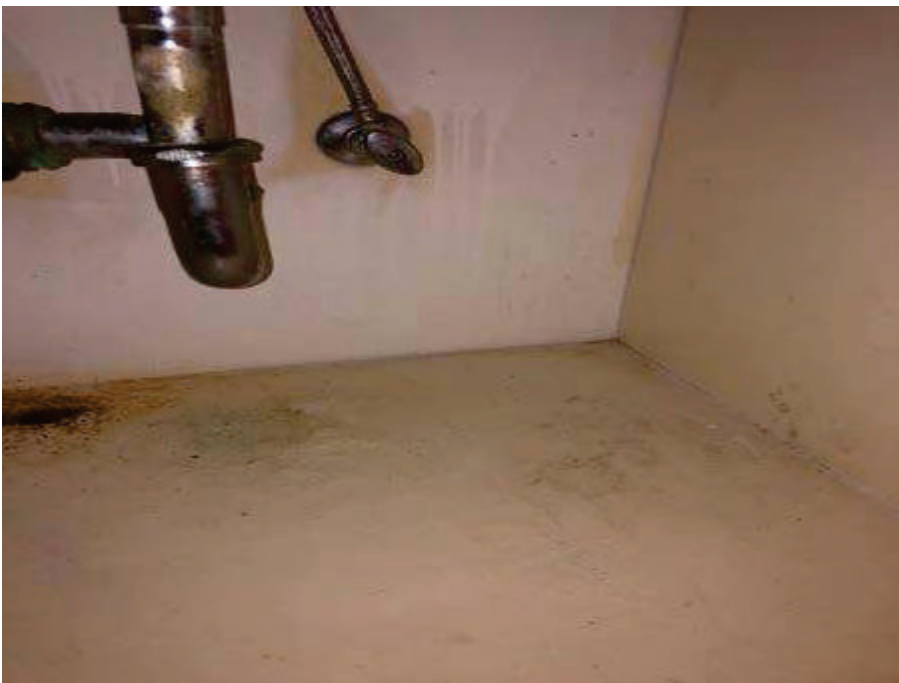
37. Marina Inn, Room 330 – View of water damage and suspect microbial growth in bathroom underneath the sink.
