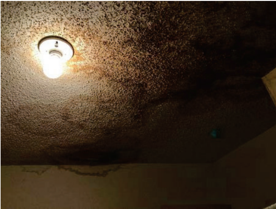
16. Marina Inn, Room 3A – View of water staining and suspect microbial growth across ASO ceiling.
