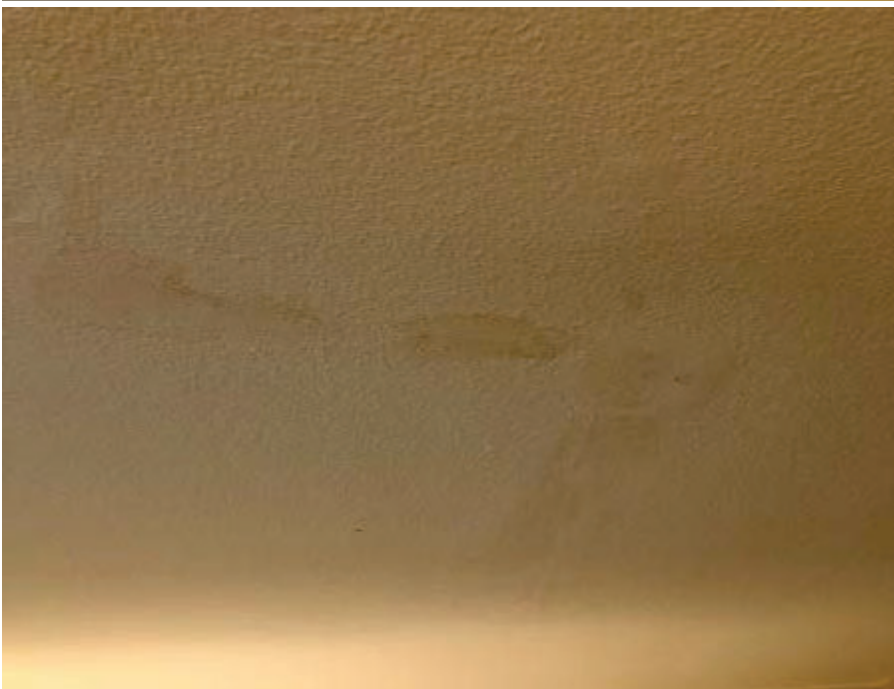
52. Marina Inn, Room 129 – View of water staining/damage on bedroom ceiling.
