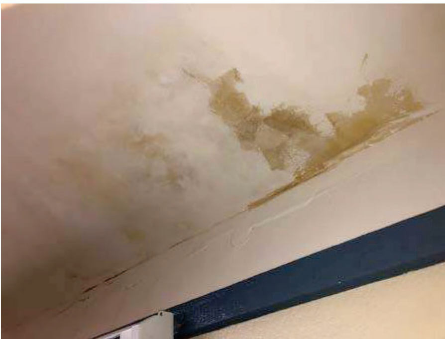
54. Marina Inn, Dana Point Room – View of water staining/damage on ceiling.
