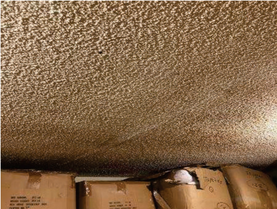
27. Marina Inn, Room 3E – View of water staining and crack in the ceiling.
