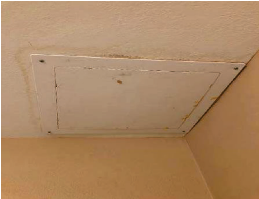
58. Marina Inn, Room 109, Office – View of visible water stains around the bathroom ceiling hatch.
