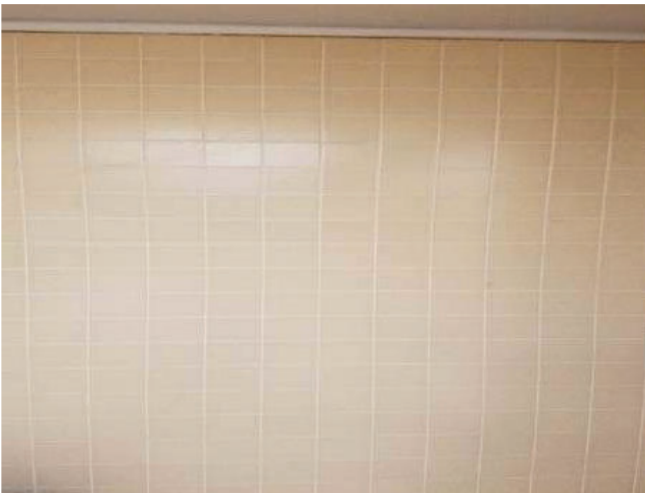
15. Building 3 – View of lead-based ceramic tile in the 1 st Floor Men's Restroom wall.
