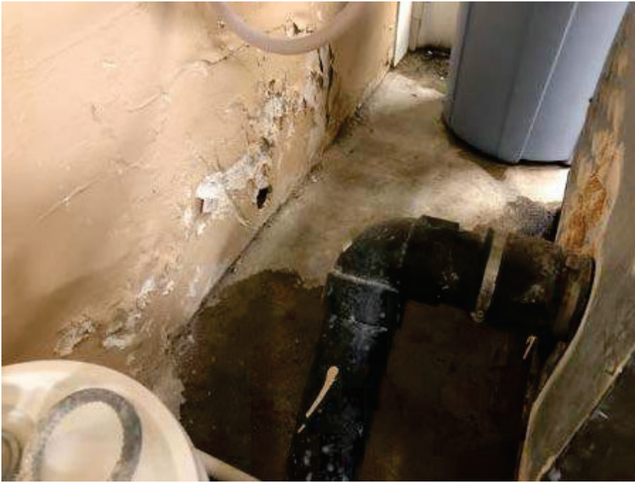
57. Marina Inn, Housekeeping – View of water staining/damage, visible water, and suspect microbial growth on East wall behind washer.
