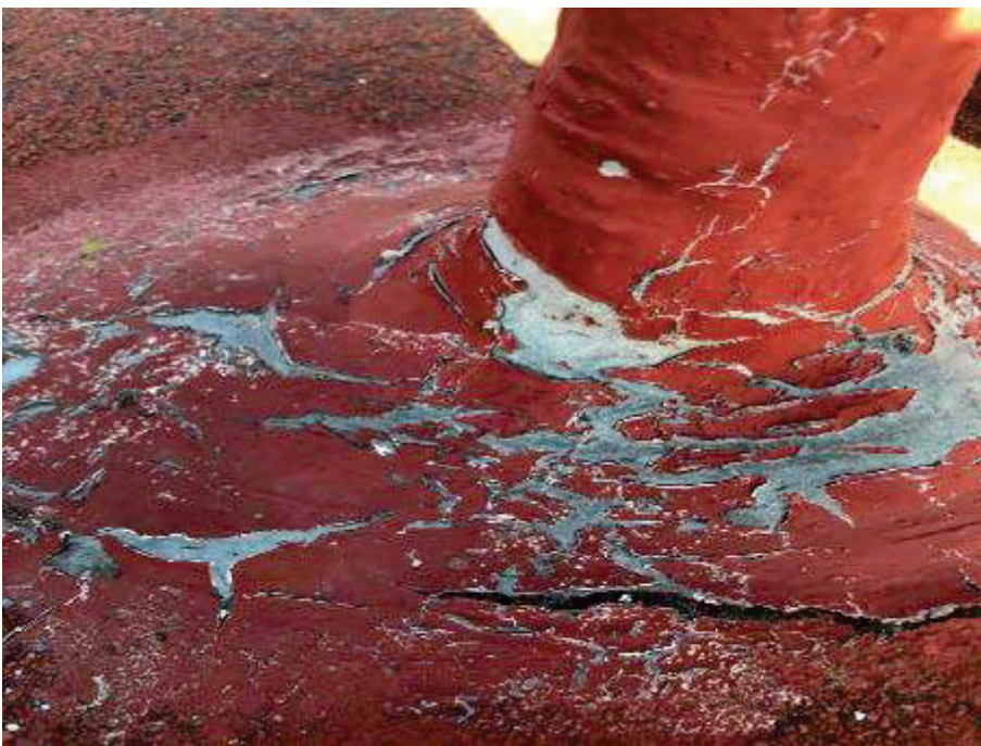
8. Marina Inn – View of ACBM red penetration mastic.
