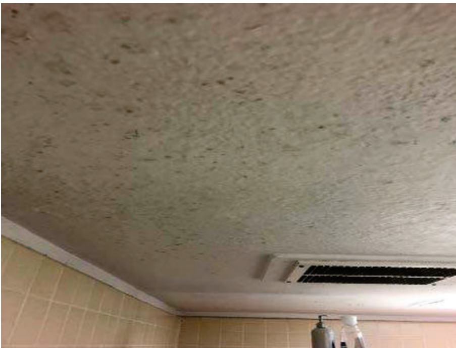
61. Building 4, Men's Restroom – View of suspect microbial growth on plaster ceiling above showers.
