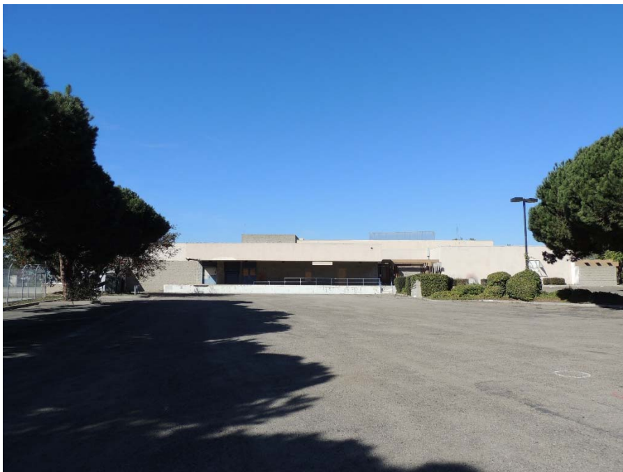
East façade, view facing west.
