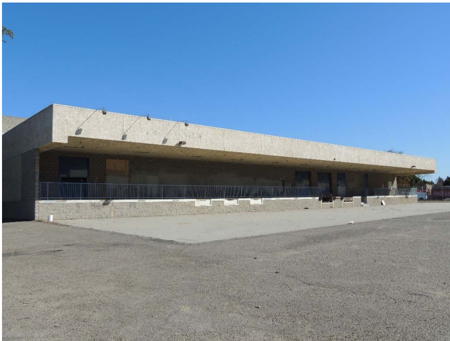
South façade, view facing northeast.
