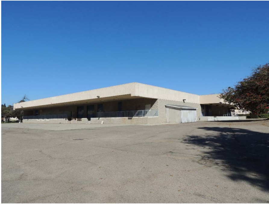
South and east façades, view facing northwest.
