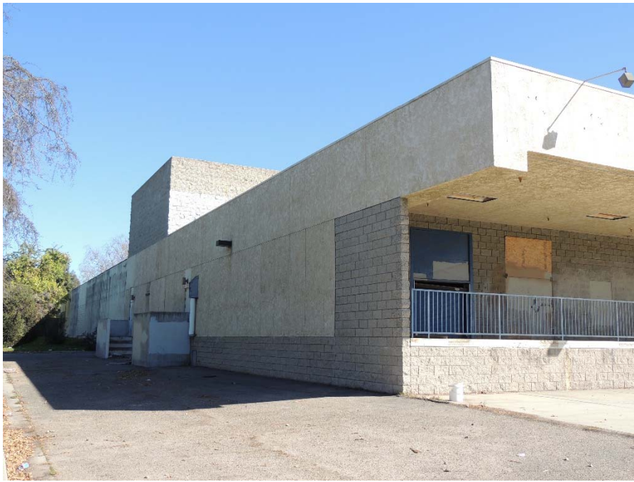
West façade, view facing northeast.
