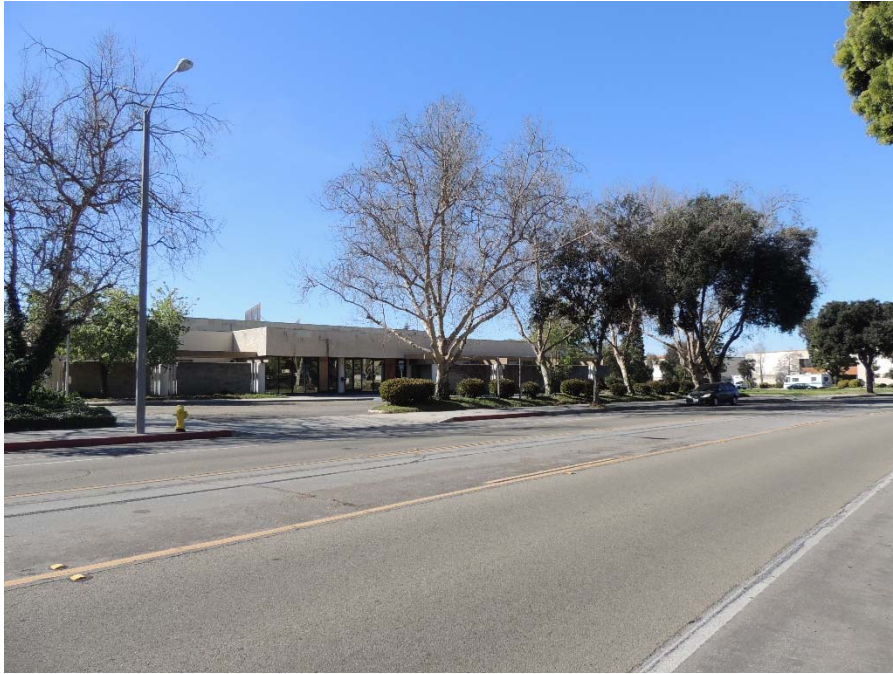
North (primary) façade, view facing southwest.
