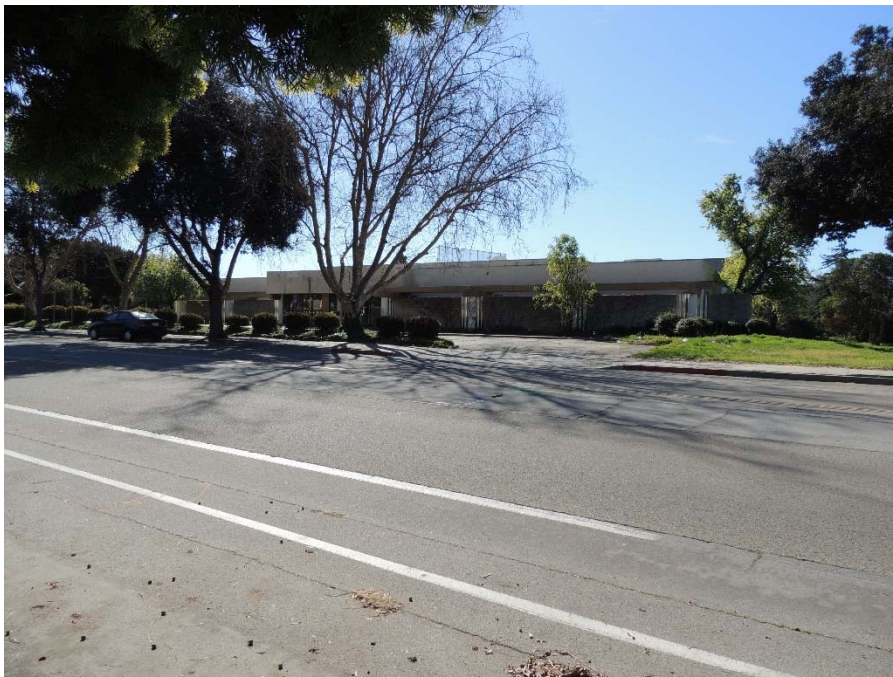
North (primary) façade, view facing southeast.
