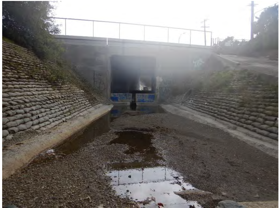
Photo 1: Upstream boundary of the Project at the Bollinger Road crossing.
