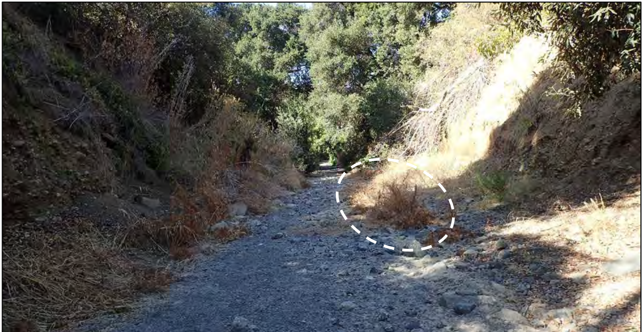
Photograph 10. Another example of a patchy vegetation growing up in the Calabazas Creek channel bed. These features are considered to be vegetated areas below the OHWM.
