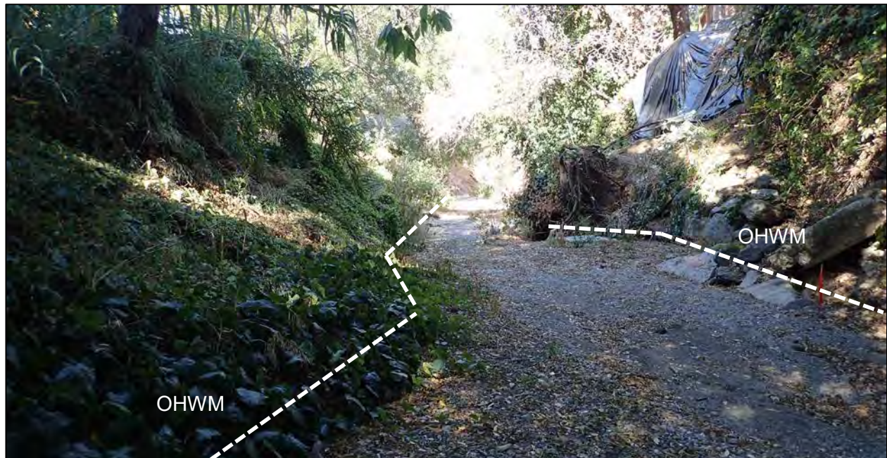
Photograph 13. An upstream (south-facing) view of Calabazas Creek at the location of a bank failure on the west bank. The collapse has narrowed the channel by approximately one foot in width. A scour hole has developed beneath the root system of the collapsed tree and the OHWM was measured on the west bank to the extent of the scouring.
