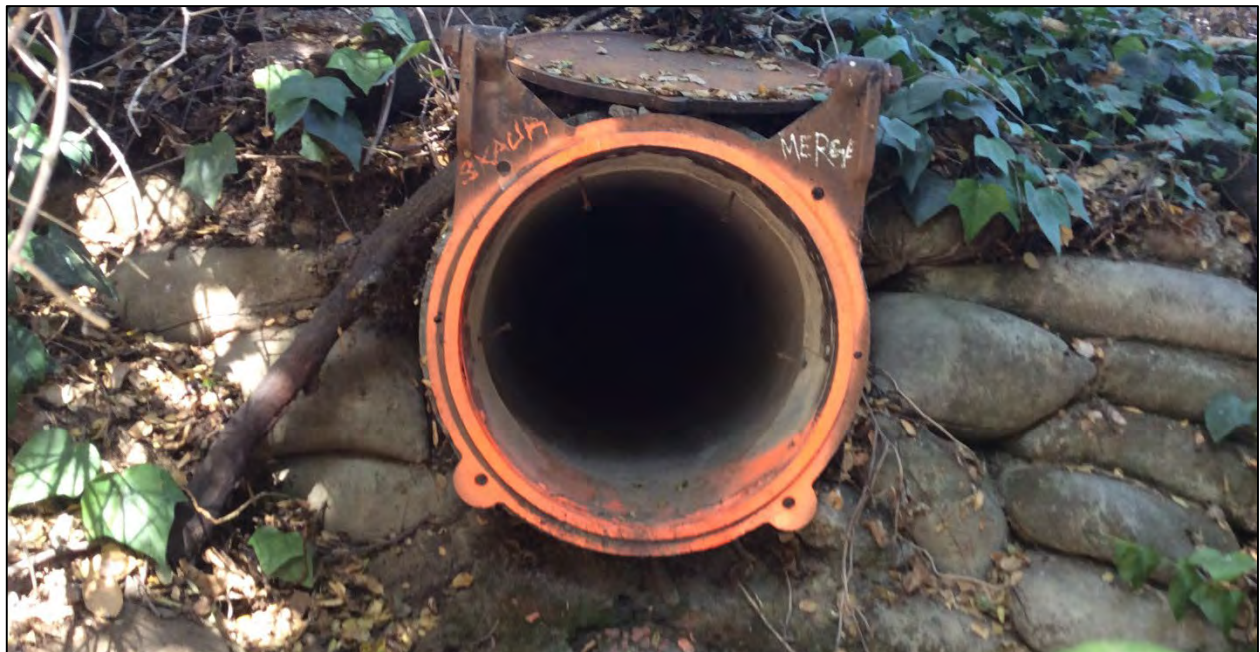
Photograph 14. A culvert outfall pipe (C3), embedded in a wall of sack-crete, empties from above the OHWM into Calabazas Creek.
