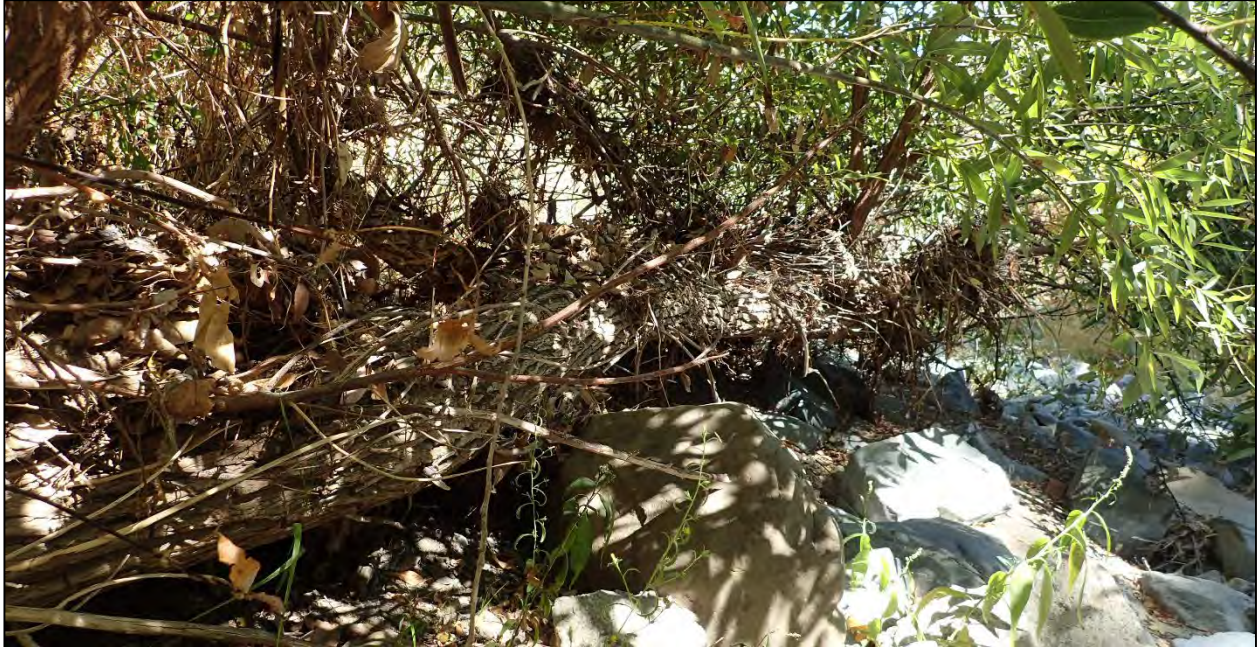
Photograph 3. West bank of Calabazas Creek at OHWM Transect 2, facing north. OHWM is evident under an overhanging willow ( Salix sp.) by a change in wrack vegetation cover that corresponds to water staining on the east bank.
