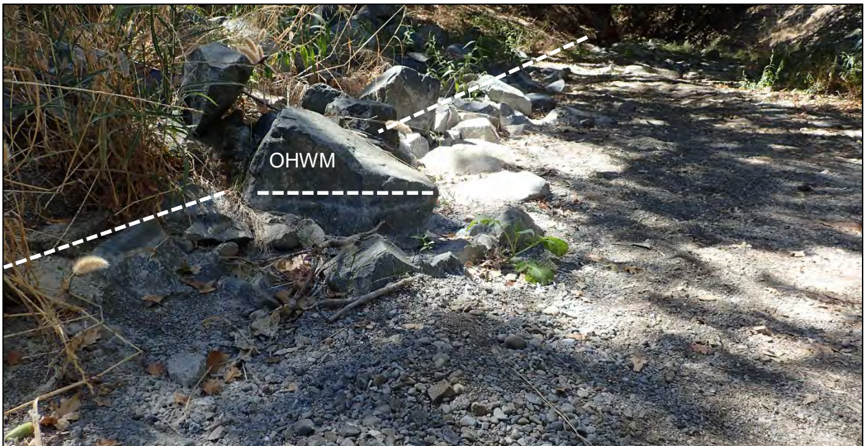
Photograph 4. East bank (facing south) of Calabazas Creek at OHWM Transect 2. OHWM is evident from a distinct water stain line on riprap placed along the bank. The sparsely vegetated gravel and coarse sand channel bed is covered in spots by a dried algal mat. Change in vegetation cover is apparent at the OHWM on the bank.
