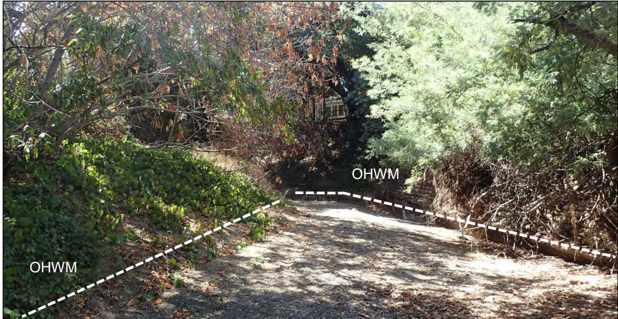
Photograph 11. Scour lines undercut a sack-crete lined bank indicating OHWM (right). On the opposite bank a break in bank slope and the change in vegetation cover marks the OHWM (left).
