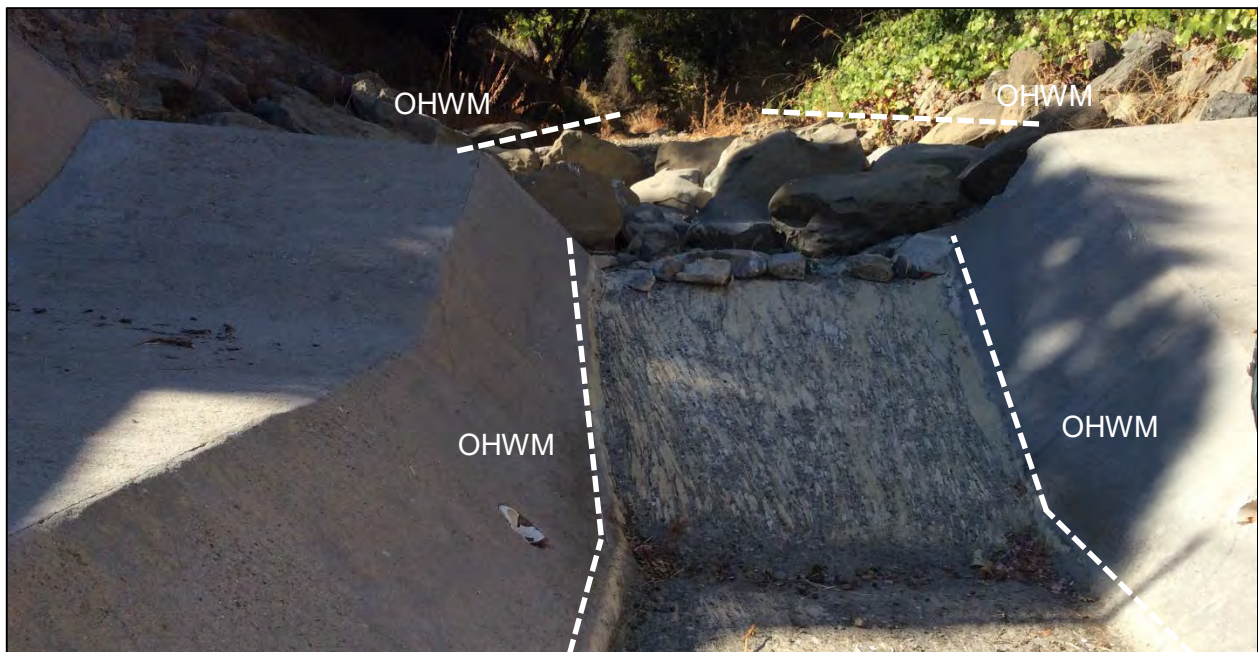
Photograph 2. Upstream (south-facing) view of Calabazas Creek channel just south of OHWM Transect 1. In this section, Calabazas Creek is contained by a cement channel flowing under Miller Avenue (top of photo). OHWM evident by water staining and algal mat in channel bed. Upstream in the earthen channel bed, change in vegetation cover is one of the OHWM indicators.
