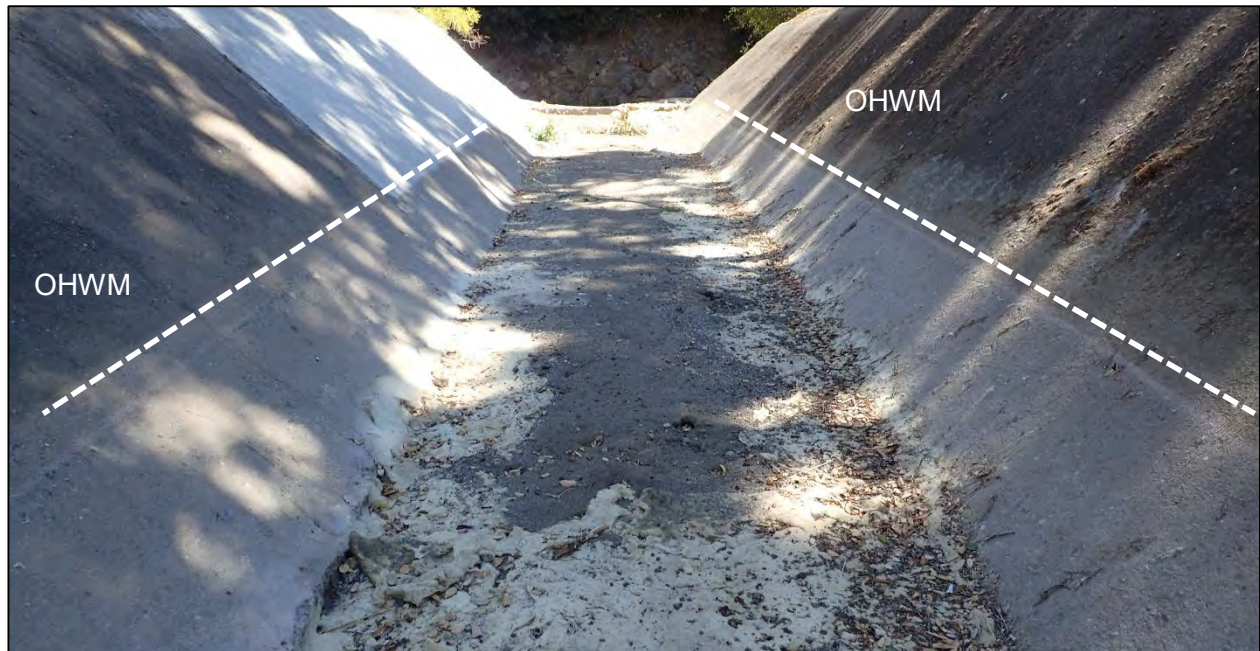
Photograph 7. Regnart Creek at OHWM Transect 3, facing east and looking downstream at the confluence of Regnart and Calabazas Creeks. Regnart Creek is a trapezoidal-shaped cement sided channel with an earthen bed. The OHWM is evident from a water stain on the cement and a change in vegetation (the absence of mosses). A dried algal mat covers much of the channel bed.
