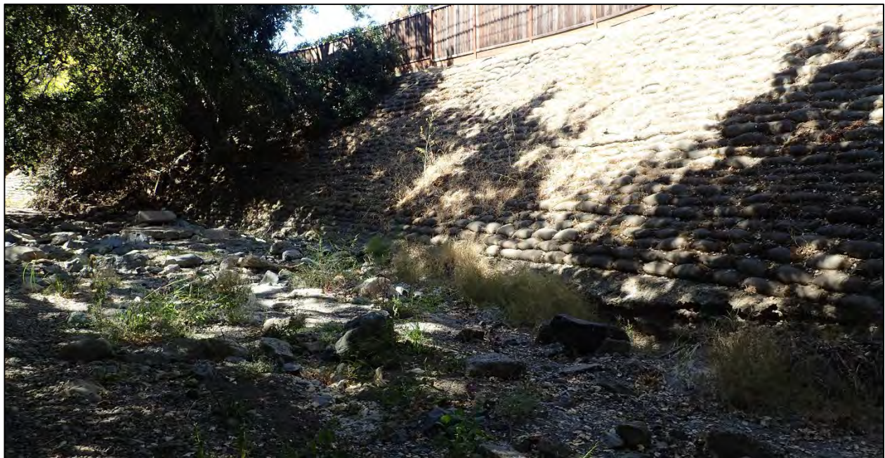
Photograph 6. Sack-crete wall stabilizing the west bank of Calabazas Creek south of OHWM Transect 2. Uninterrupted lines of residential fences (top) stretch along both sides of the creek just beyond the top of bank for the entirety of the survey area.
