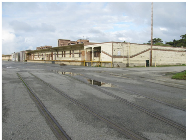
PHOTO 3.4: View from southwest corner of site facing northeast. Note rail junction in foreground.
