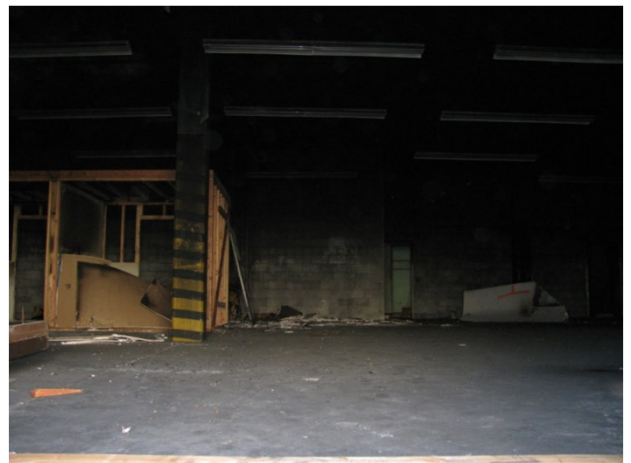
PHOTO 4.5: Interior of Building 2071 and Fire Department training area.
