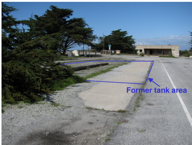
PHOTO 4.3: View of Former tank area facing north
