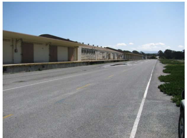
PHOTO 4.4: View of 1 st avenue and former rail yard, facing south.
