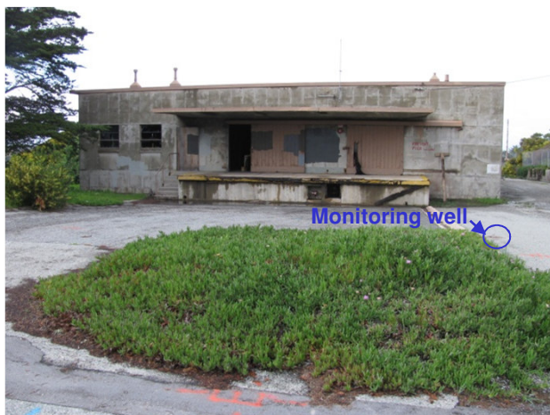
PHOTO 3.1: View of Building 2071 facing north from 8 th Street. Note location of nearby monitoring well.
