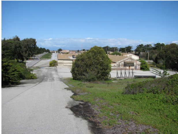
PHOTO 4.1: View of south edge of site, facing north
