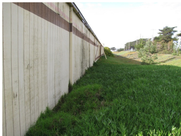
PHOTO 3.6: View of east side of site. Note buildings to left are storage buildings east of Quartermaster Ave.
