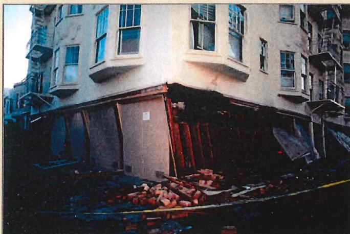
Lack of adequate shear walls on the garage level exacerbated damage to this building at the corner of Beach and Divisadero in the Marina District, San Francisco, during the October 1989 Loma Prieta earthquake.
