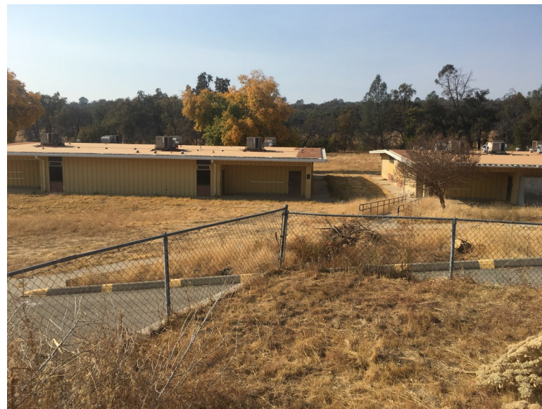
View from driveway looking west toward existing classrooms to be demolished.
