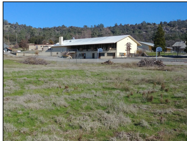
Looking northeast toward existing cafeteria to be demolished from southern portion of the Project site.
