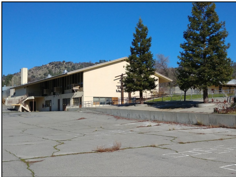
Center of site looking northwest toward existing cafeteria to be demolished.
