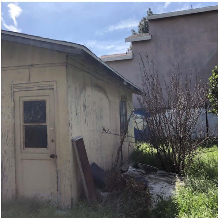
Photo 7 – View of northwest building corner of Granny Unit looking south
