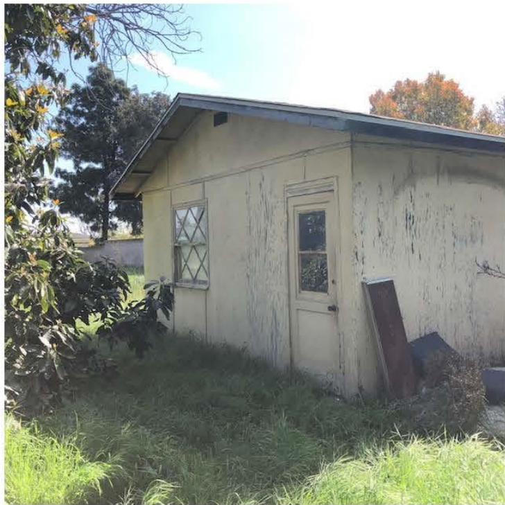
Photo 6 – View of front entrance of Granny Unit looking to southeast parcel corner
