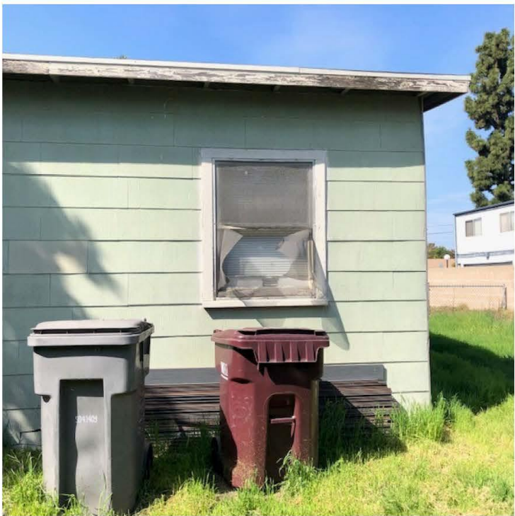
Photo 8 – View of southeast building corner of 305 N Mountain View St looking west
