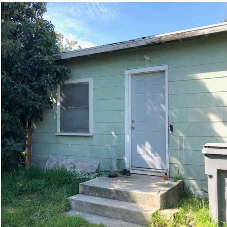
Photo 9 – View of rear entrance of 305 N Mountain View St
