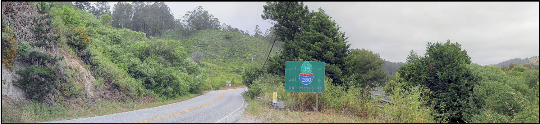
Photograph 3a. Existing Conditions, Looking East
