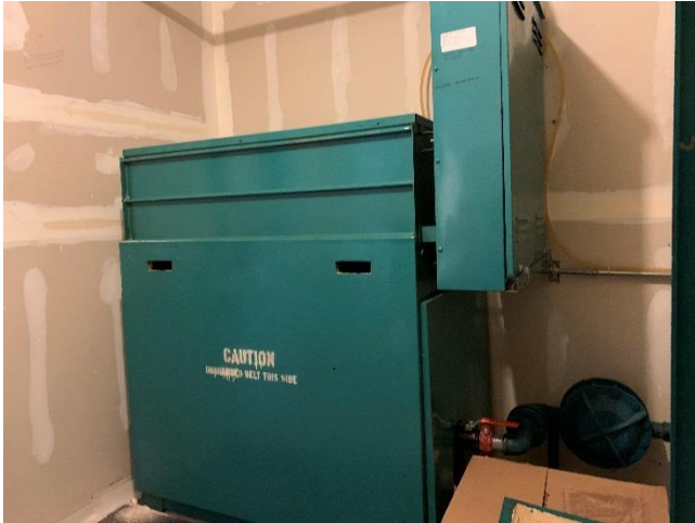
Photo 1: Hydraulic system for elevator in the Orange County Museum of Art tenant space.
