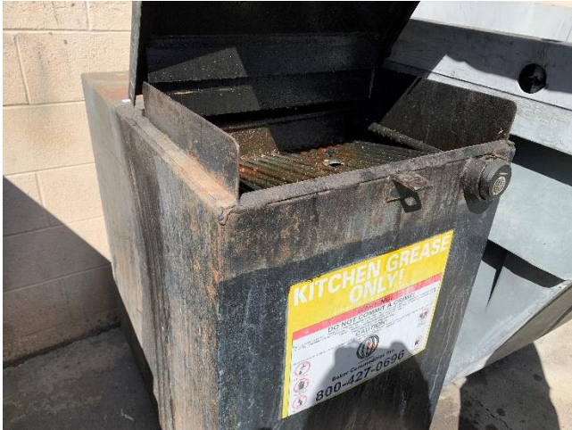
Photo 19: Kitchen grease collector at outdoor trash collection area.
