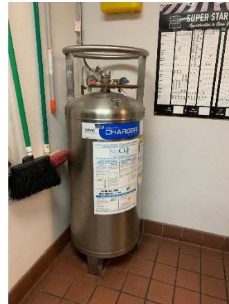
Photo 12: Liquid carbon dioxide tank at restaurant tenant space.
