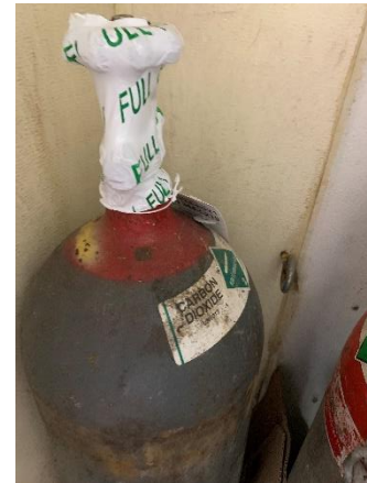
Photo 16: Carbon dioxide cylinder in restaurant tenant space.
