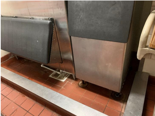
Photo 7: Floor drain in restaurant tenant space.
