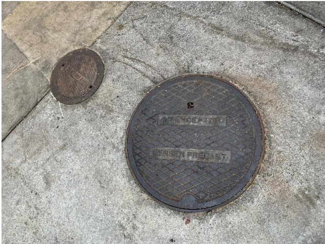
Photo 11: Grease interceptor at exterior of restaurant tenant space.
