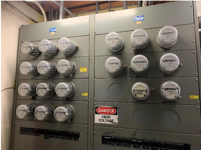
Photo 21: Electrical meter for different tenant spaces.
