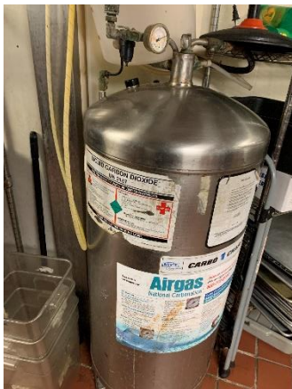
Photo 17: Liquid carbon dioxide cylinder in restaurant tenant space.
