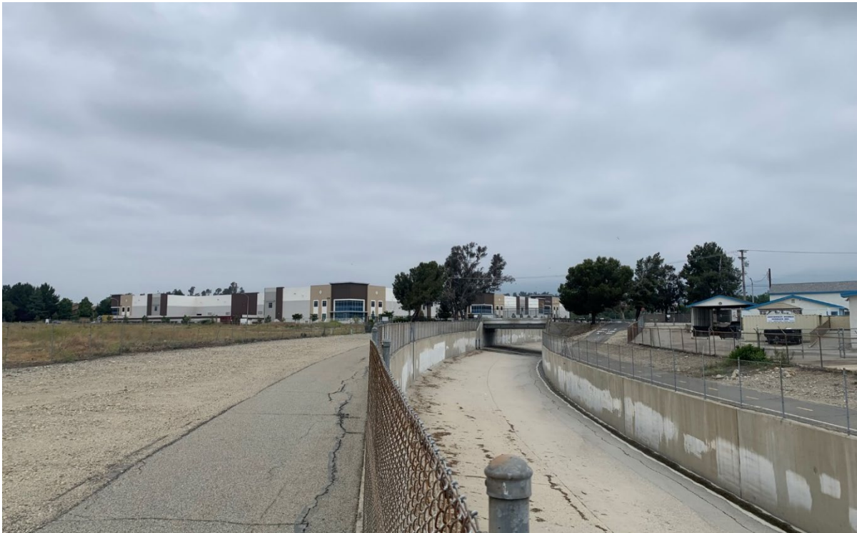
Photograph 4: North facing view of Cucamonga Creek along the northeastern boundary of the project site.
