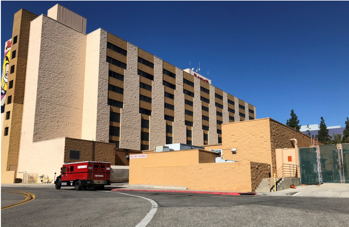
Figure 5 View of Marriott Hotel Buildings from Avon Street, Facing Northwest
