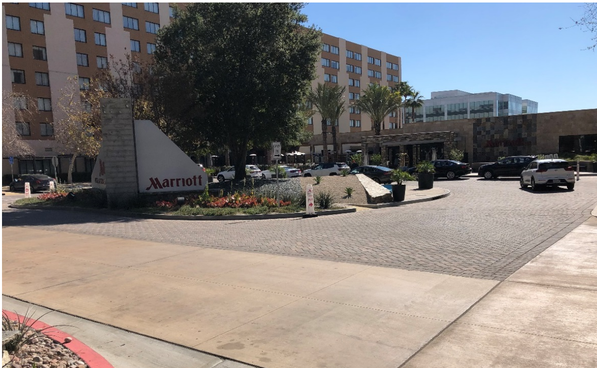
Figure 3 Overview of Western Portion of Project Site, Facing Southwest
