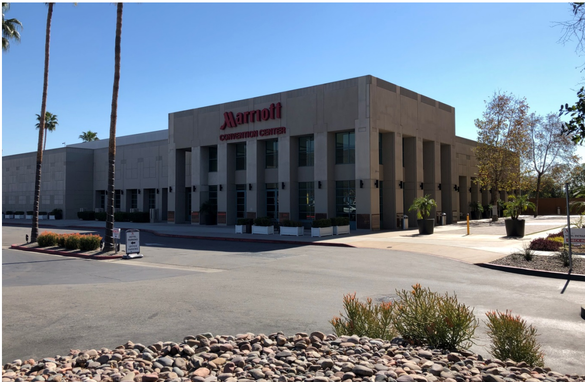
Figure 6 View of Marriott Convention Center Building, Facing Southeast
