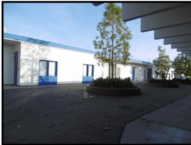
PHOTO 3: View of the Administration Building. View to the southeast.
