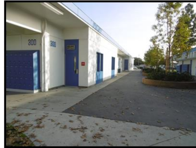
PHOTO 2: View of the Administration Building. View to the south.
