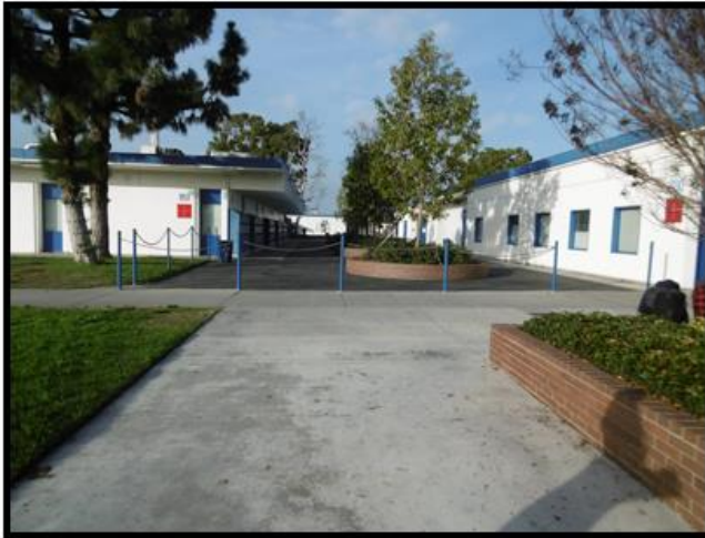
PHOTO 5: View of the area between the Administration Building and the adjacent Classroom building. View to the north.
