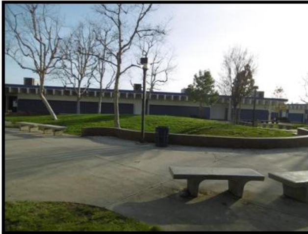
PHOTO 1: View of the Administration Building and landscaped grass area. View to the southeast.
