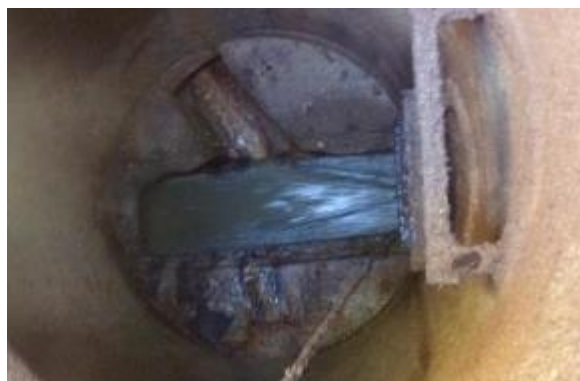
Manhole Before Install
