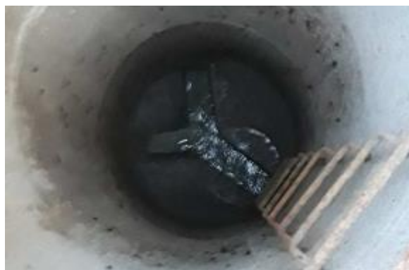
Manhole Before Install
