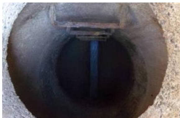
Manhole Before Install
