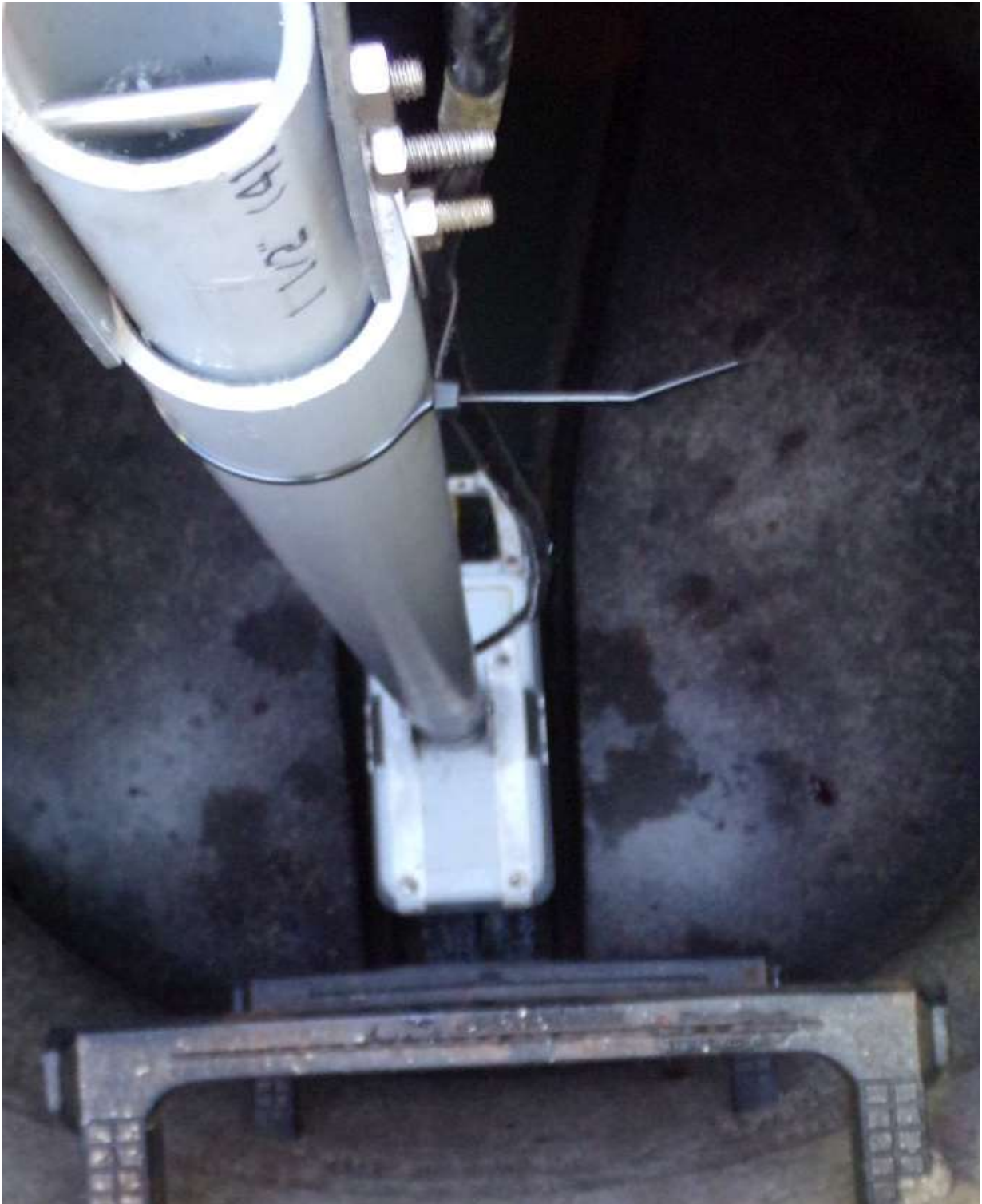
Figure above: The Nordstrom MH provided access to an 8-in sewer line, which entered from the north and discharged to the southeast. Gas levels were good (well within OSHA acceptable limits: O_2=20.9\% ; LEL, H_2S & CO=0 ). The flow monitoring equipment was set to monitor the downstream pipe as it provided the best hydraulics. Follow up on this installation confirmed equipment calibration.
