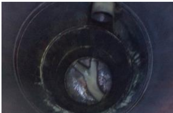
Manhole Before Install
