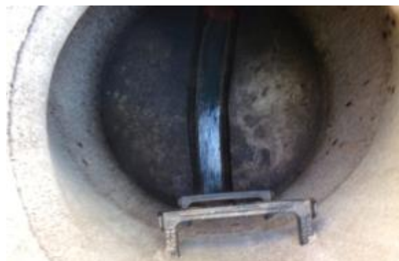
Manhole Before Install
