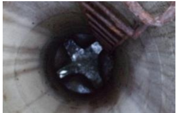
Manhole Before Install
