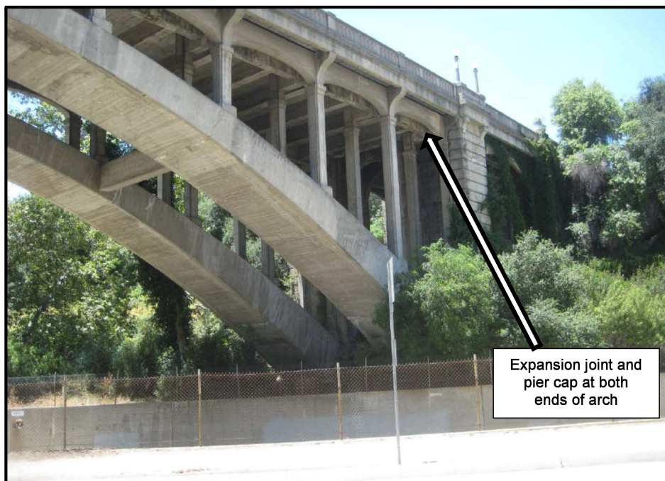
Annotated view of the bridge showing locations of proposed work, view facing west. Source: Dokken Engineering (2018).
