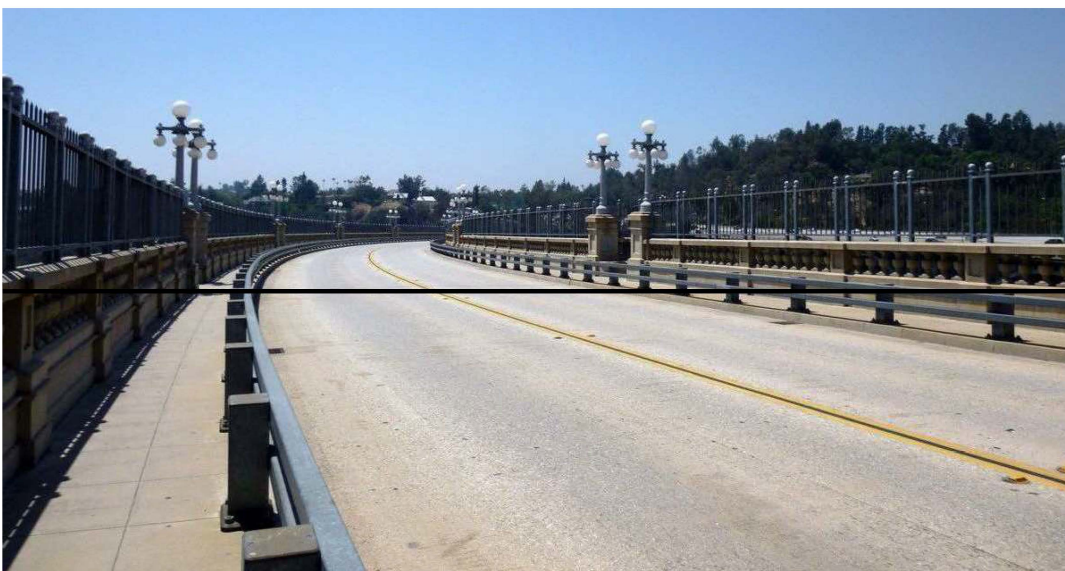
Image showing a view of the Colorado Street Bridge crash barrier. A similar barrier is proposed to be added to the Holly Street Bridge
