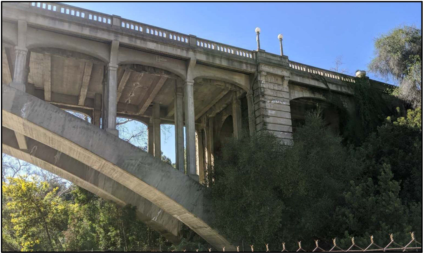
The Holly Street Bridge spandrel columns, view facing south. Source: Dokken Engineering (2020).
