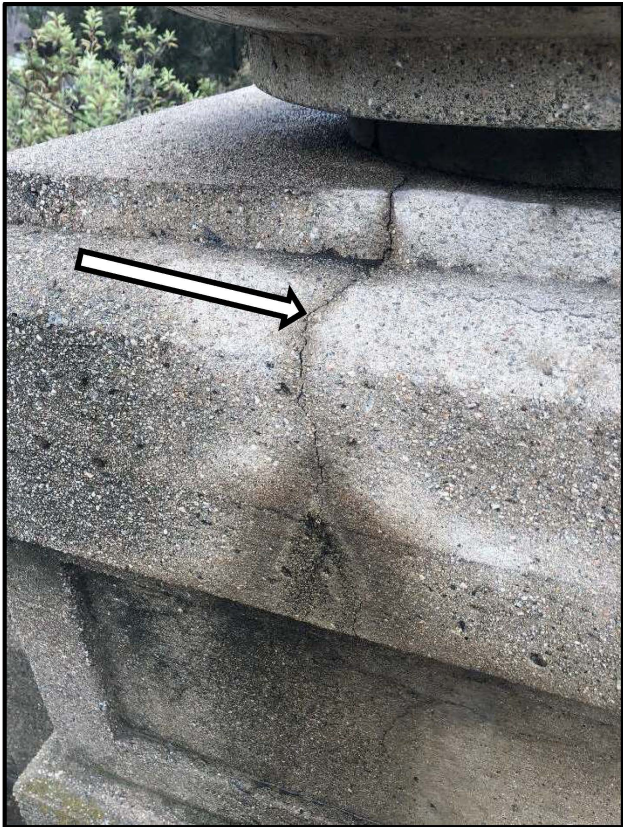
Image showing typical cracking on the Holly Street Bridge. Source: GPA Consulting (2019).
