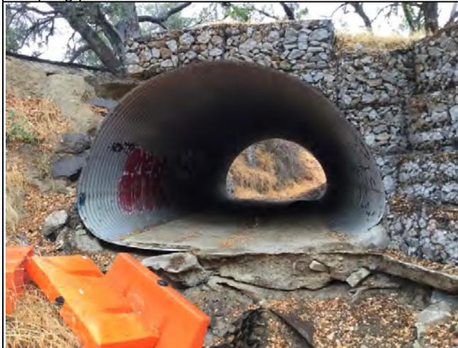
Photo 3. Photo of Waycross Rd. Culvert from downstream. Note bank / road collapse in upper left of photograph.
