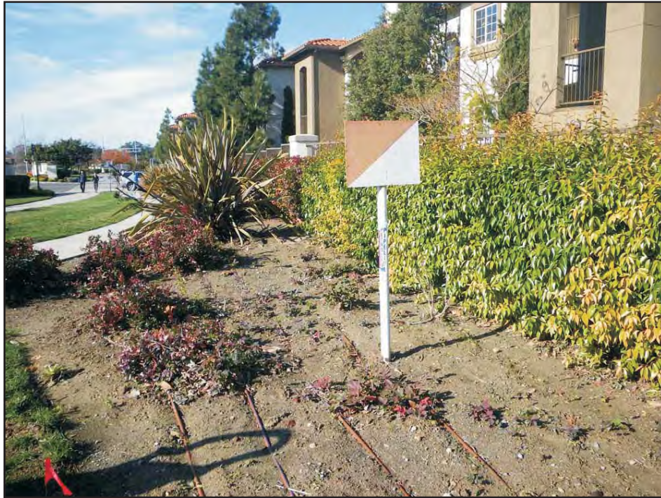
Photo 5 - View west along Chevron pipeline alignment on north side of Hilltop Drive, north of project site.
