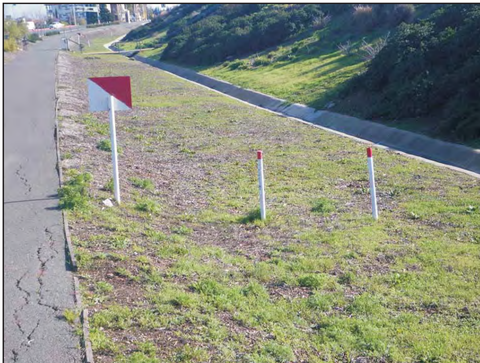
Photo 6 - View east along Chevron pipeline alignment on south side of Hilltop Drive, northwest of project site.
