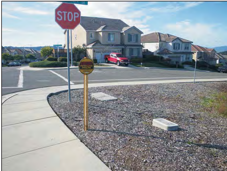
Photo 8 - View southwest toward Kinder-Morgan pipeline alignment at intersection of Park Ridge Drive and Wood Glen Drive, southwest of project site.
