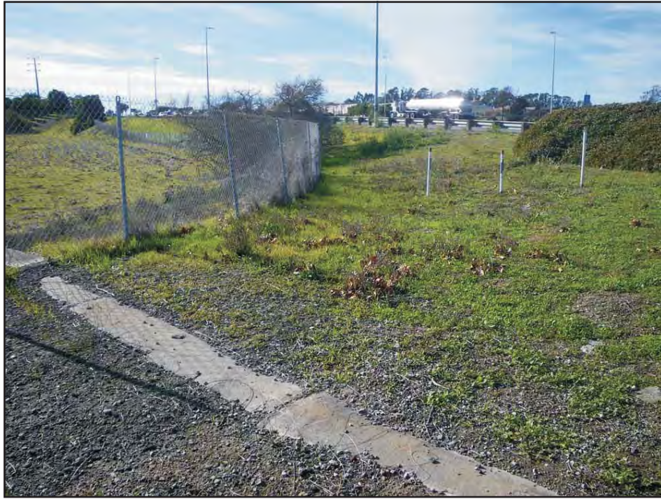
Photo 3 - View southwest toward Chevron pipeline alignment near northwest corner of project site; project site at left; Richmond Parkway at right.
