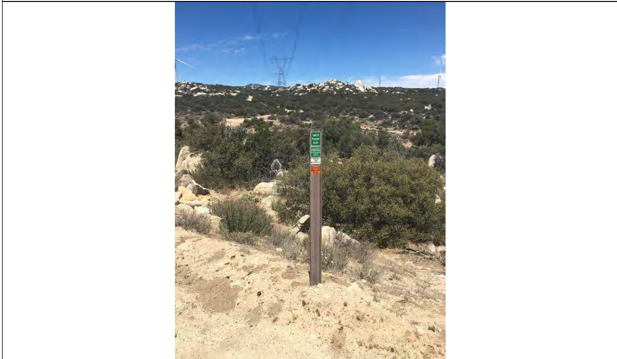
Photo 35. Utility powerline that runs across the northern section of the property. Post is at the edge of a crane pad for one of the stands. Bottom of post mentions herbicides in use.
