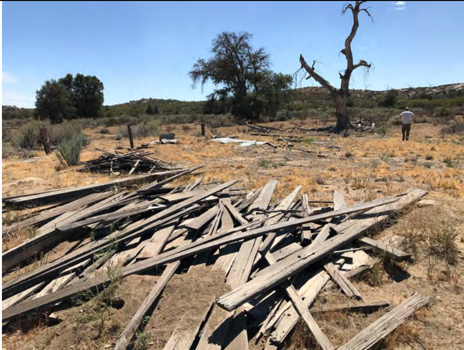
Photo 43. Remnants of a possible collapsed structure 700 feet south of the cattle yard. Wood planks, cut granite blocks, and metal sheet roofing are present. No tanks or other utilities found.
