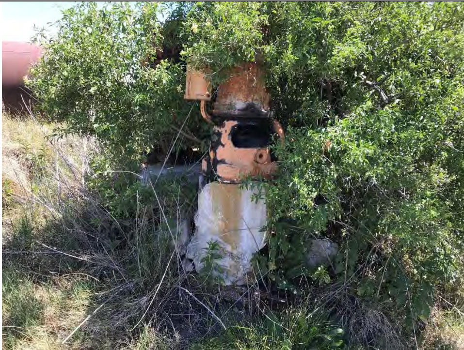
Photo 25. Groundwater well covered in vegetation with AST in the background.
