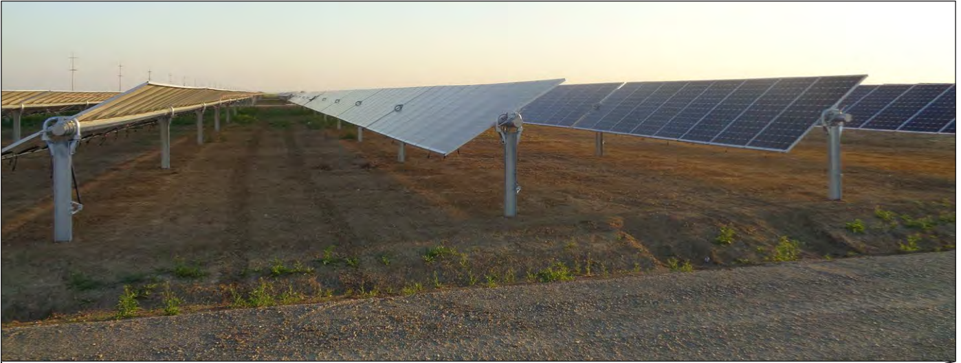
Solar PV Modules on Horizontal Trackers
