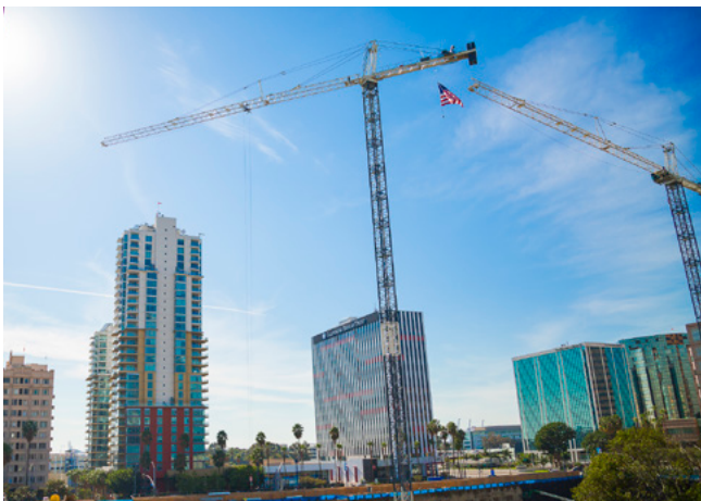
Construction of city hall
