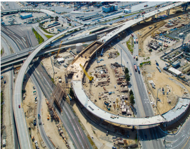
Freeway interchange in Long Beach
