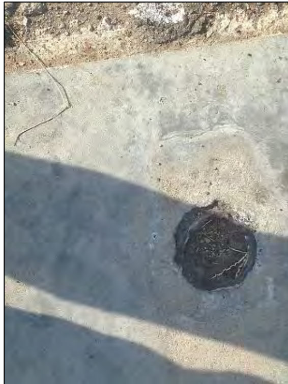
Photograph 4: Possible previous boring location in concrete patch at 2211 Merced St.
