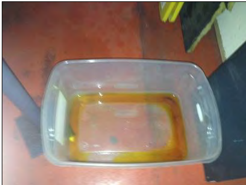
Photograph 6: Oil in plastic pan beneath elevator motor in FCFCU building
