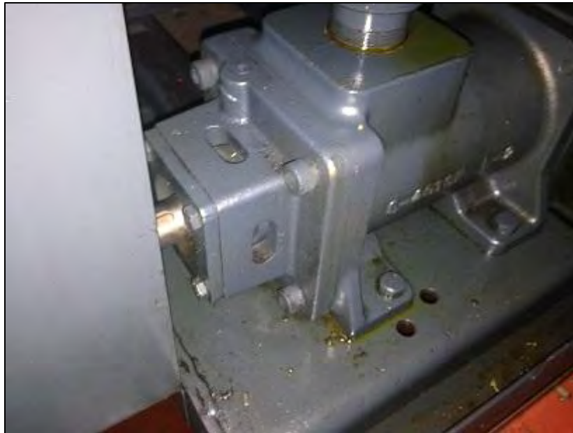
Photograph 5: Oil on exterior of elevator motor in FCFCU building
