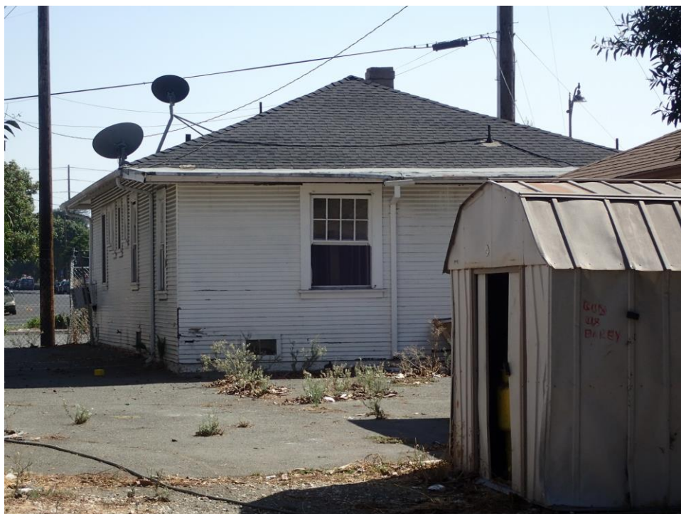
Rear elevation, viewed facing south.
