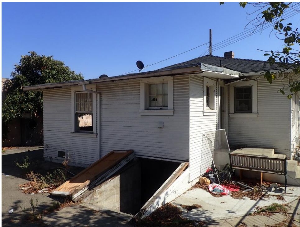
Rear elevation, viewed facing southeast.
