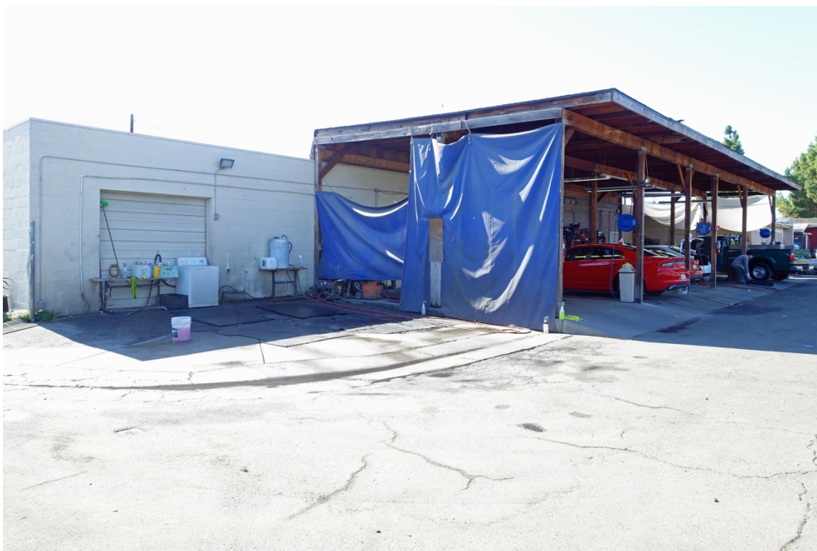
Figure 2. North elevation. 1433-1463 El Camino Real. October 2018.
