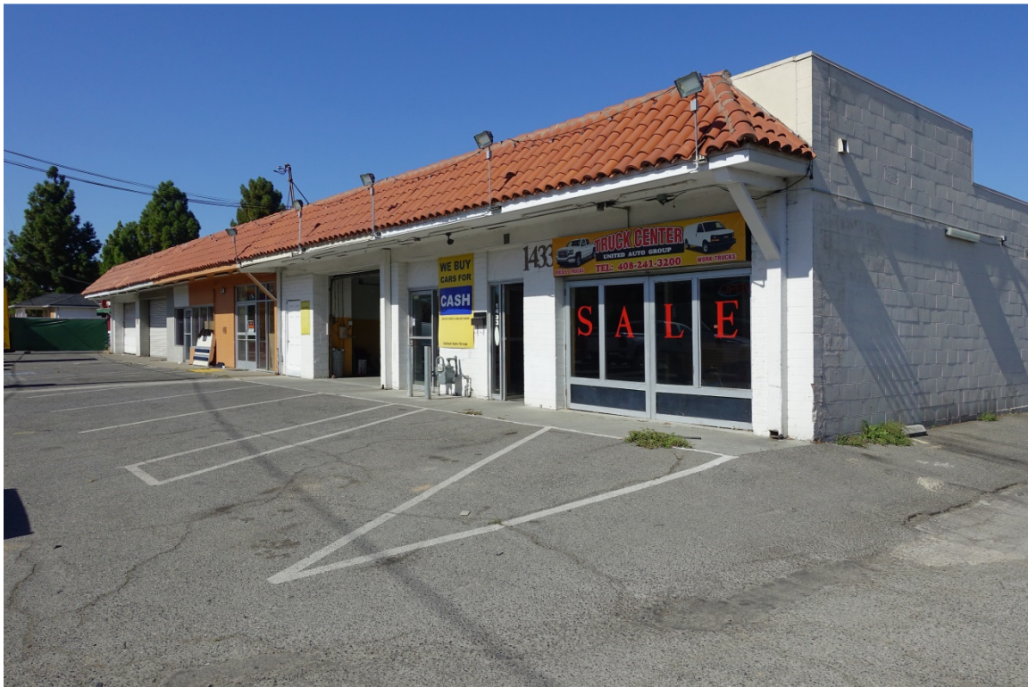
Figure 1. South elevation. 1433-1463 El Camino Real. October 2018.
