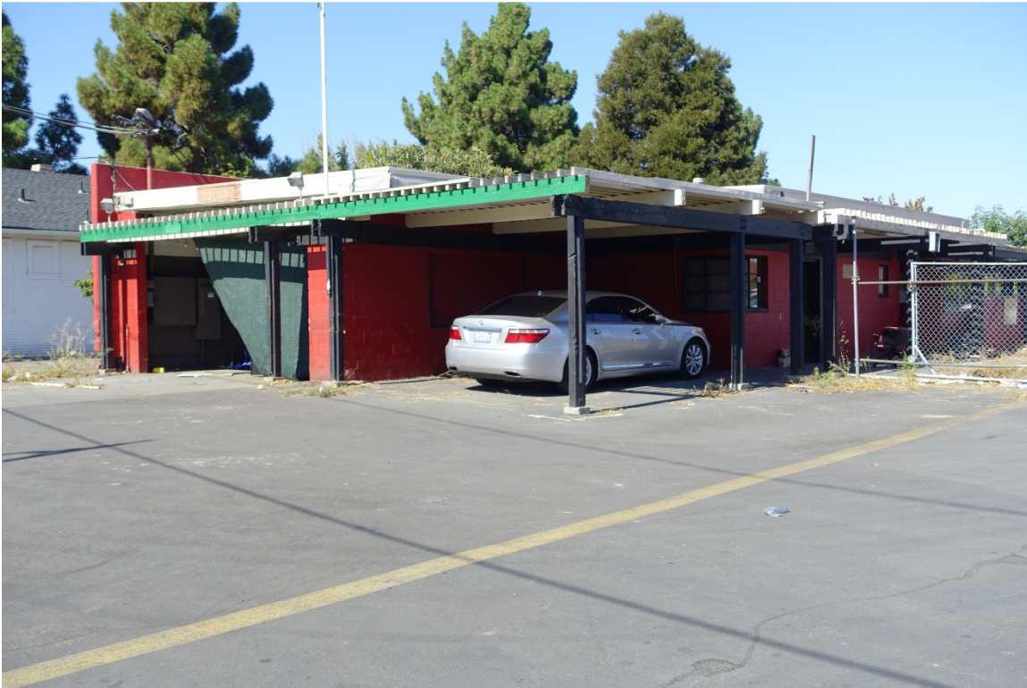
Figure 1. South and east elevations. 1483 El Camino Real. October 2018.
