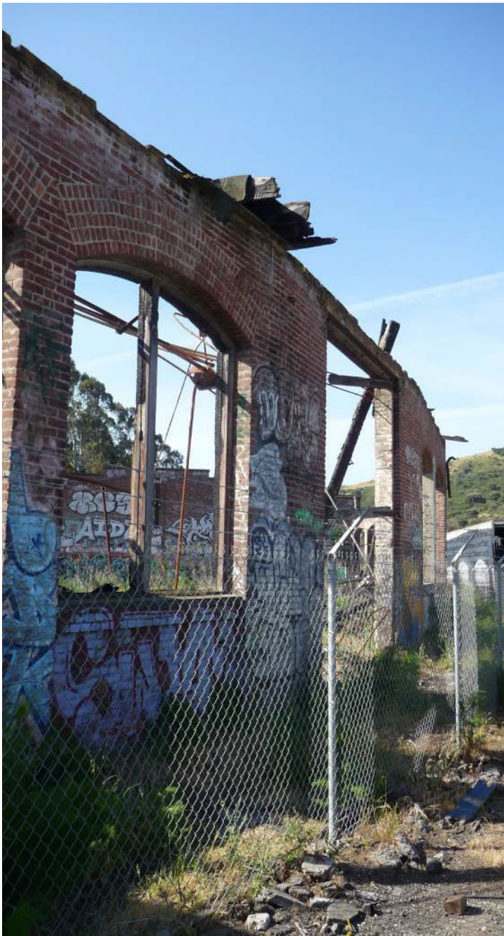
Figure 12: The only oversize opening in the burned south area has no leaf and minimal window material remains.
