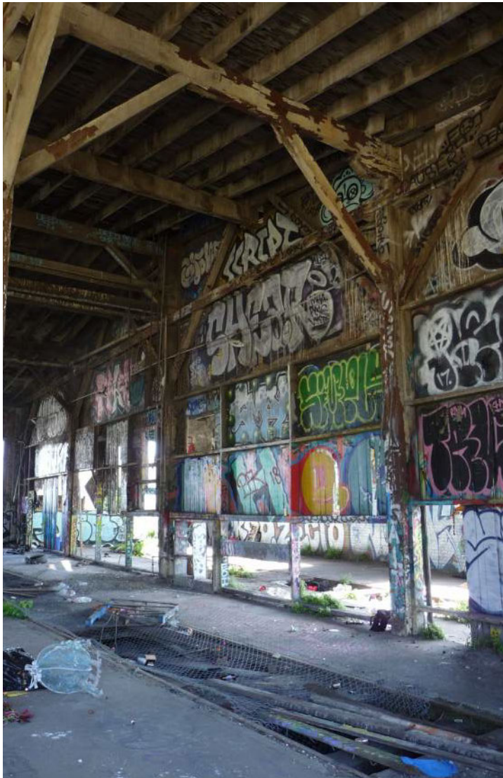
Figure 24: The wood panel wall between two bays. Sections are lost.
