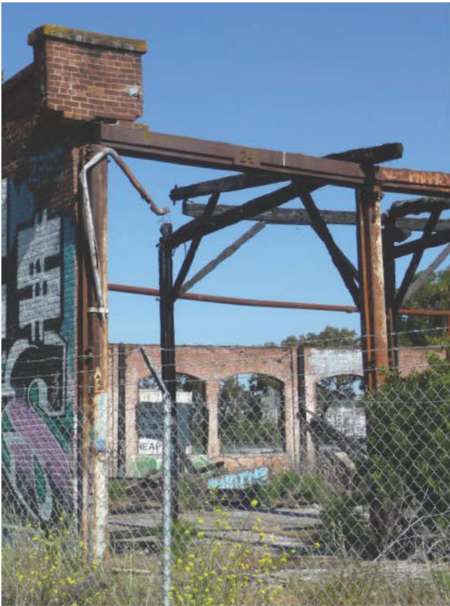
Figure 29: The steel structure provided the inner circumference support.
