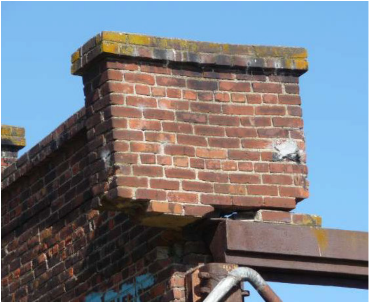
Figure 8: At the south end firewall, the inner wall's end parapet is detaching from its supports.
