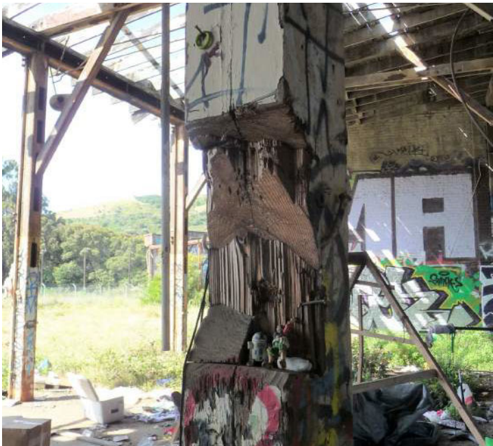
Figure 25: Some posts have sections cut out of them.
