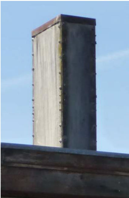
Figure 15: (left, above) Sheet metal smokestacks.
