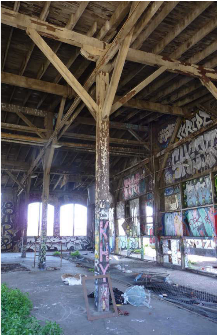
Figure 23: The wood post and beam structure with knee braces.
