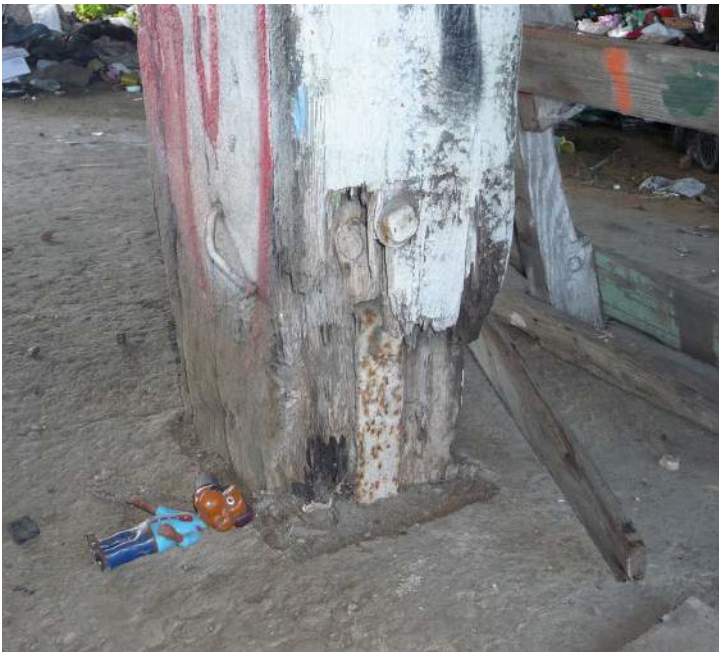
Figure 26: Insect damage where the posts are bolted to the slab.
