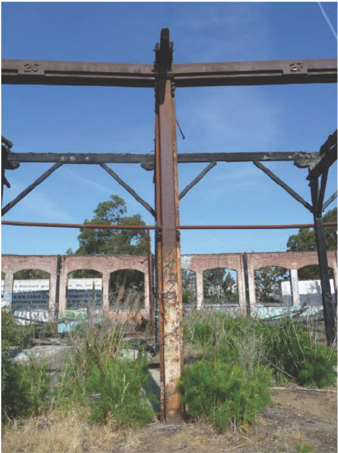
Figure 30: Expected surface corrosion and paint are evident.
