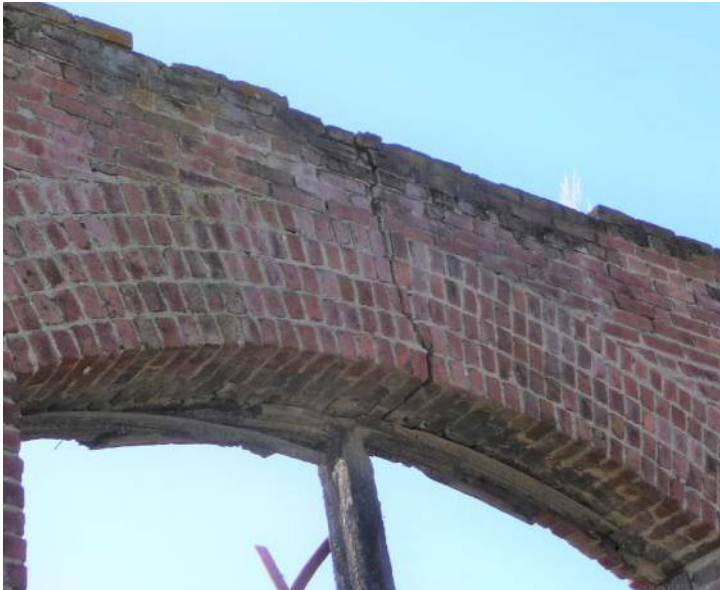
Figure 7: There is cracking through some arches over openings.
