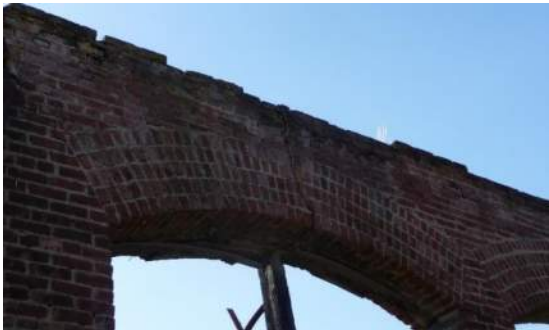
Figure 3: Cracked lintel to receive shoring.
