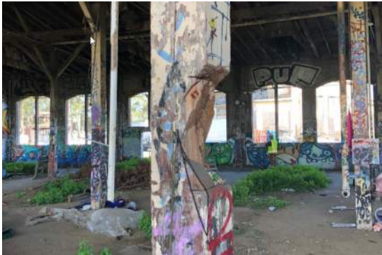
Figure 2: Notched wood column to receive shoring.
