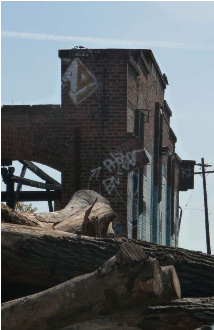
Figure 9: The south end firewall is leaning out from the rest of the Roundhouse. Whether it is a function of settlement or simply itself is tilting is unknown.
