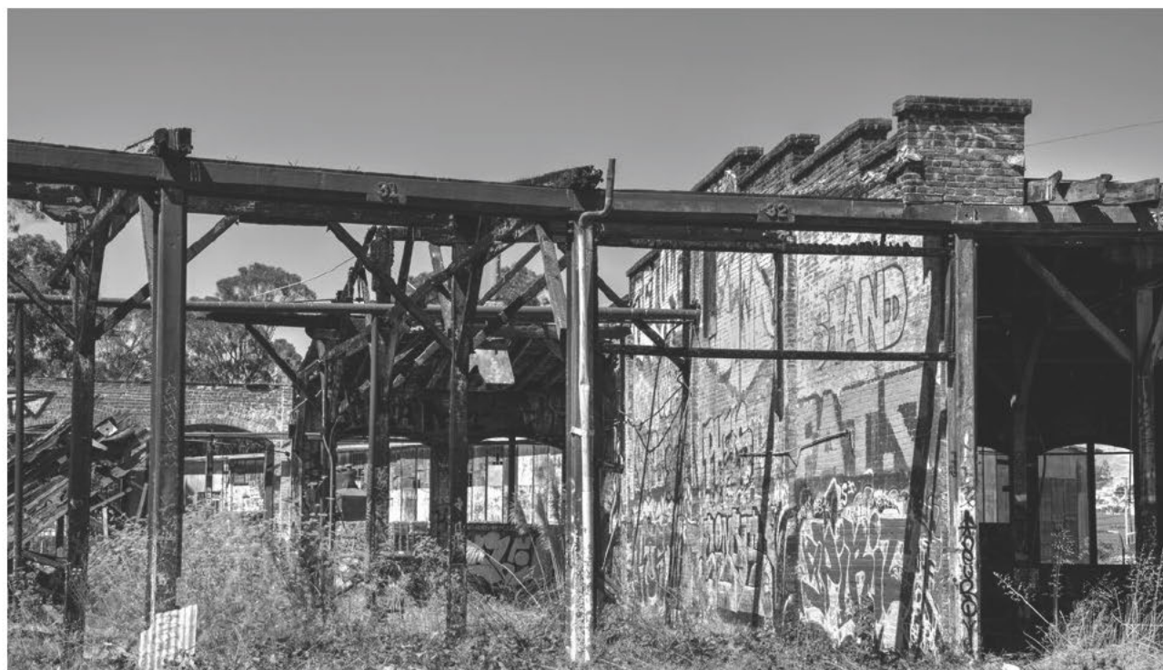
Photo 17 Cast Iron Stall Posts with lintels/stall numbers
