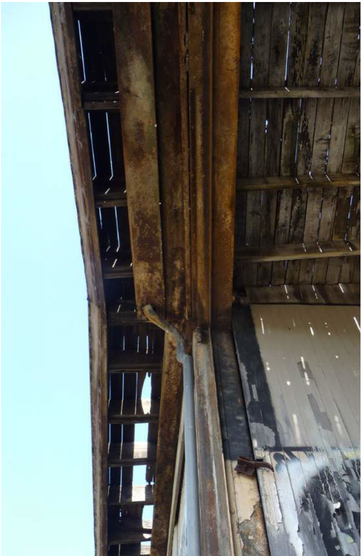
Figure 22: Missing roofing resulting in visible gaps through roof.
