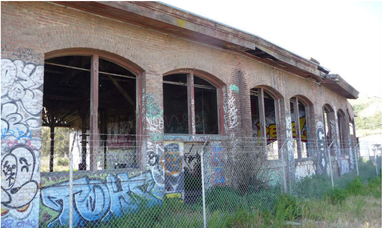
Figure 6: Graffiti along the outer circumference is obvious. Some staining at down spout and roof leaks are also apparent.
