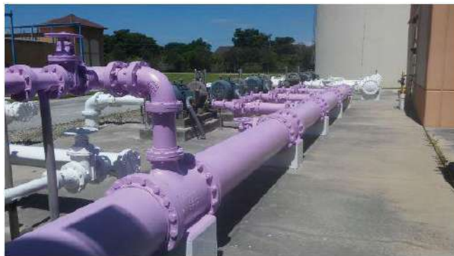
Purple pipe is used to designate reclaimed water and separate it from potable water. (Image Source: Brown and Caldwell)
