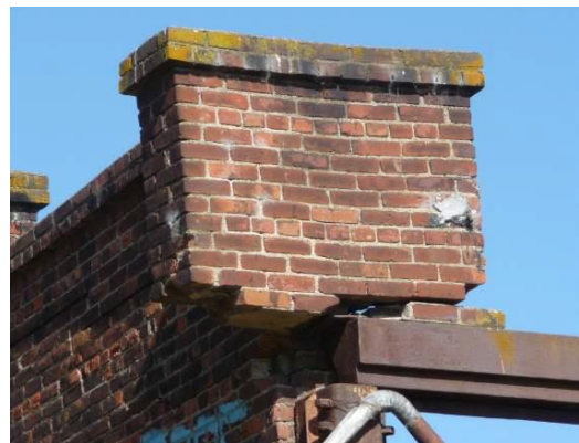
At the south end firewall, the inner wall's end parapet is detaching from its supports.
