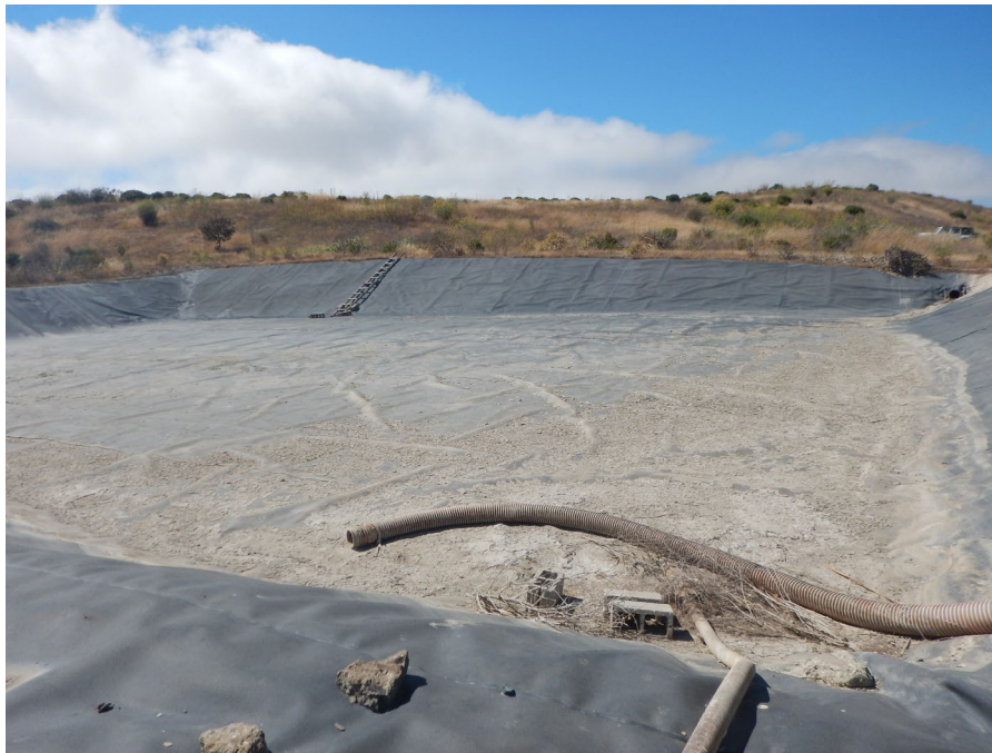
Figure 35 Constructed Basin (CB)
