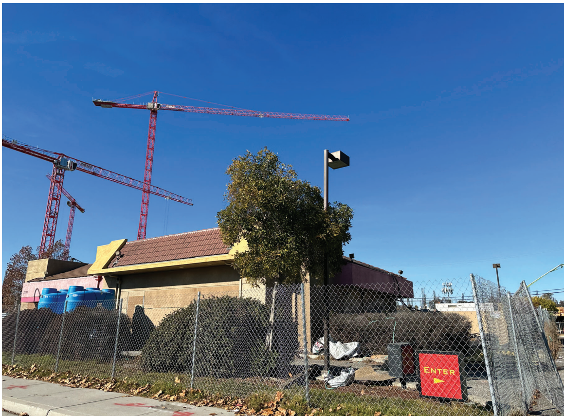
Photo 8: View of on-site construction from Tasman Drive looking northwest.
