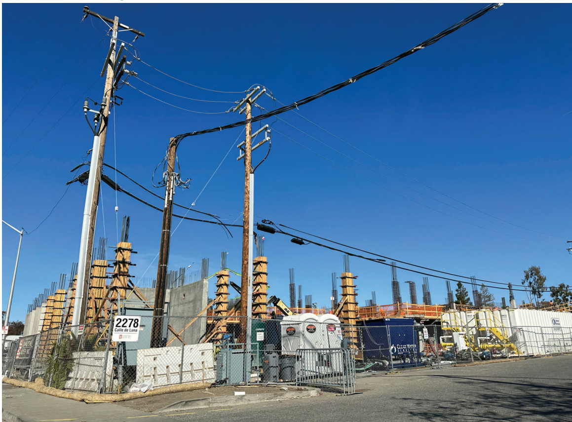
Photo 6: View of on-site construction from Calle Del Sol looking northeast.
