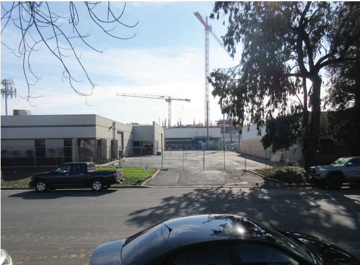
Photo 2: View of on-site construction from Calle Del Mundo looking south.
