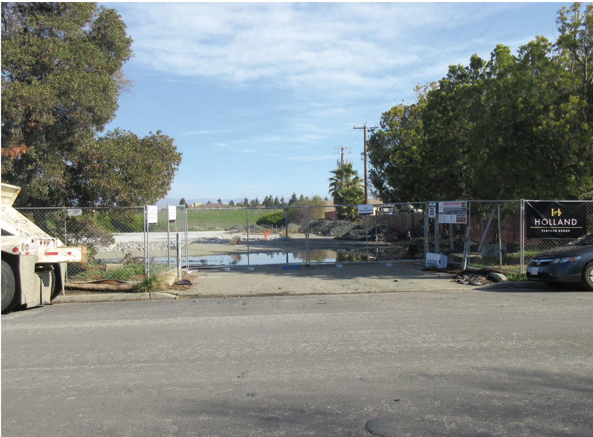
Photo 4: View of on-site construction from Calle Del Mundo looking northeast.
