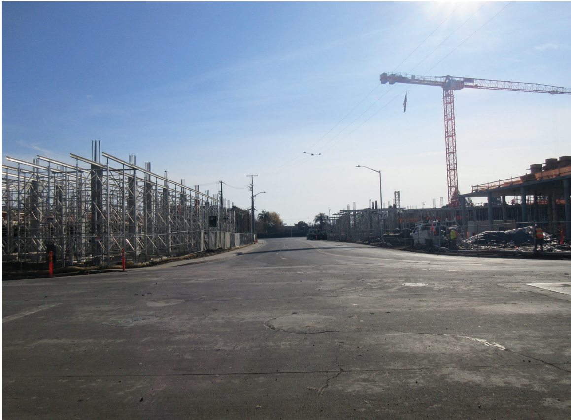
Photo 5: View of on-site construction from the intersection of Calle De Luna and Calle Del Sol looking south.
