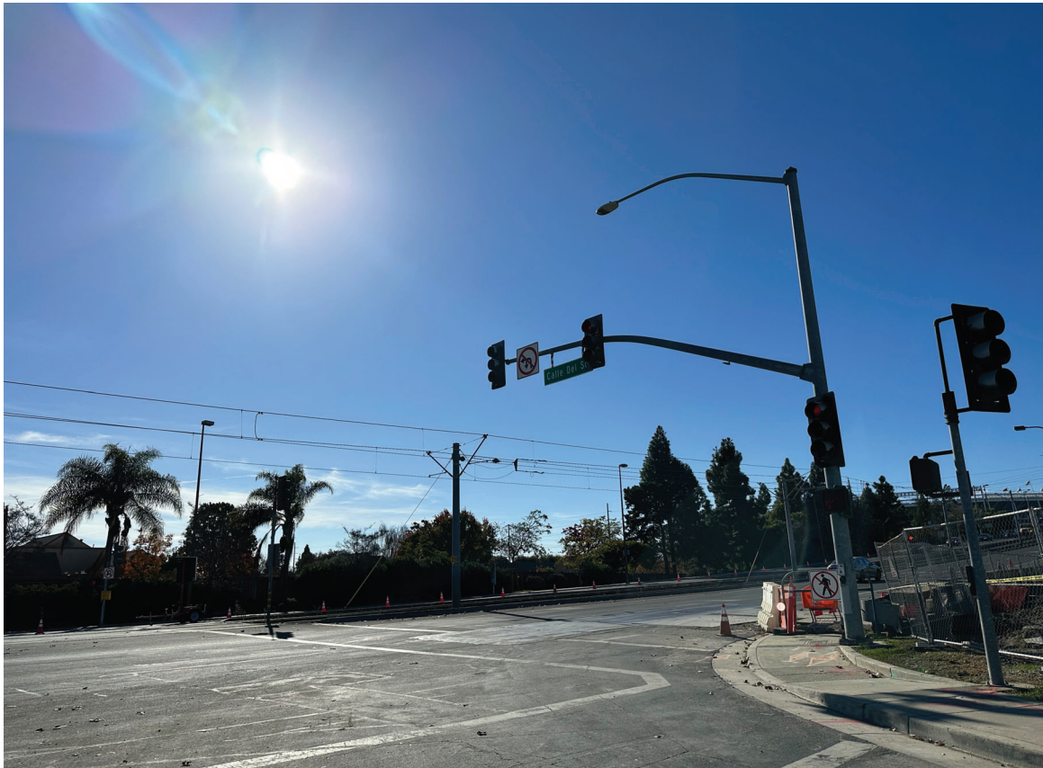
Photo 7: View from Calle Del Sol and Tasman Drive intersection looking southwest.
