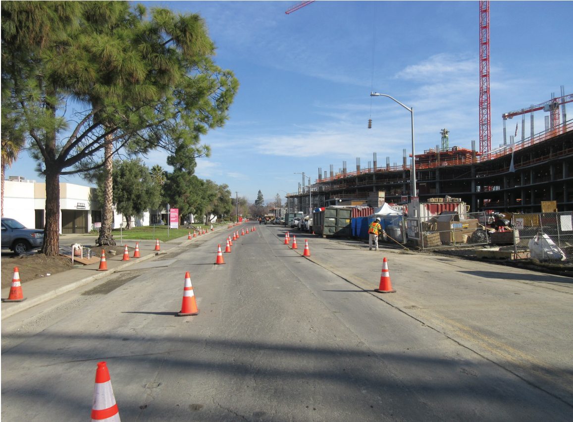
Photo 9: View of Calle De Luna from west side of project site looking northeast.
