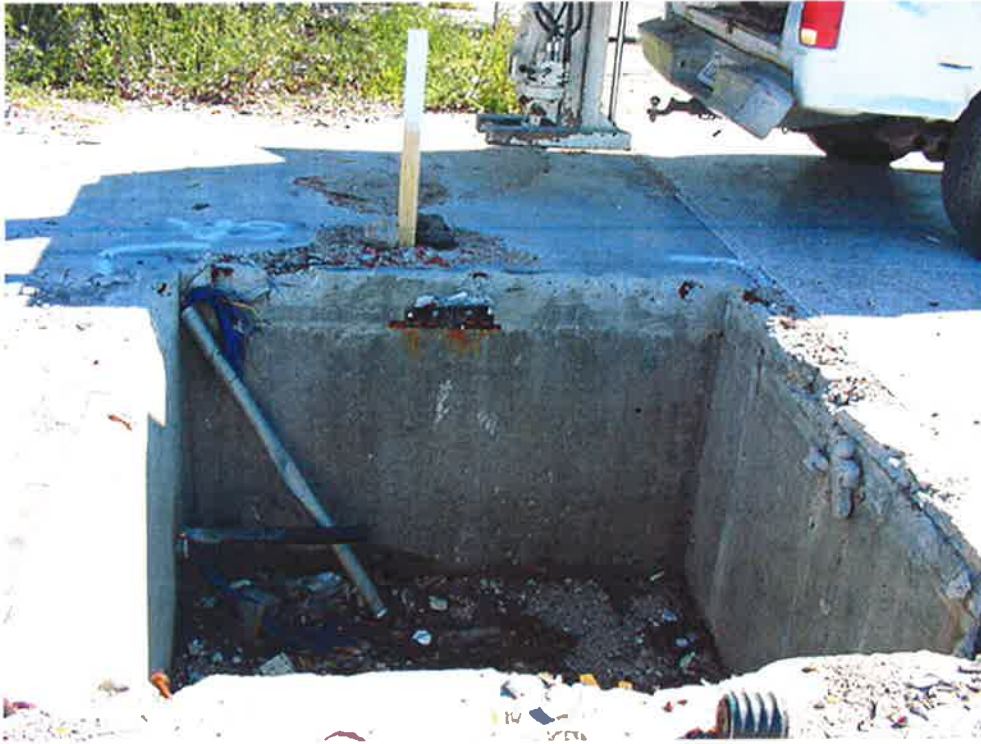
Hydraulic elevator pit with soil boring location shown.
