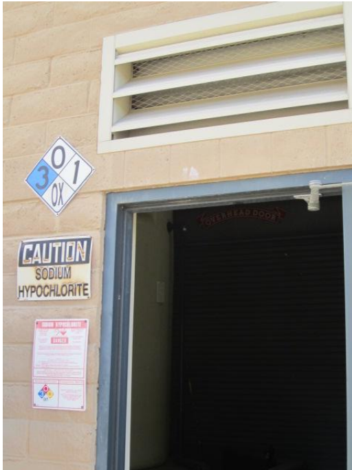
Photo 13. Sodium hypochlorite feed room entrance
