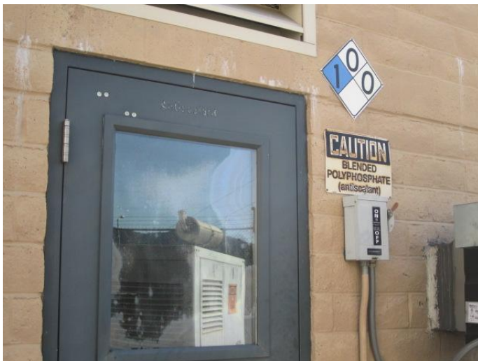
Photo 12. Anti-scalant feed room entrance
