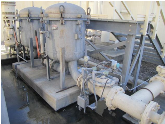
Photo 9. Backwash/recycle equipment
