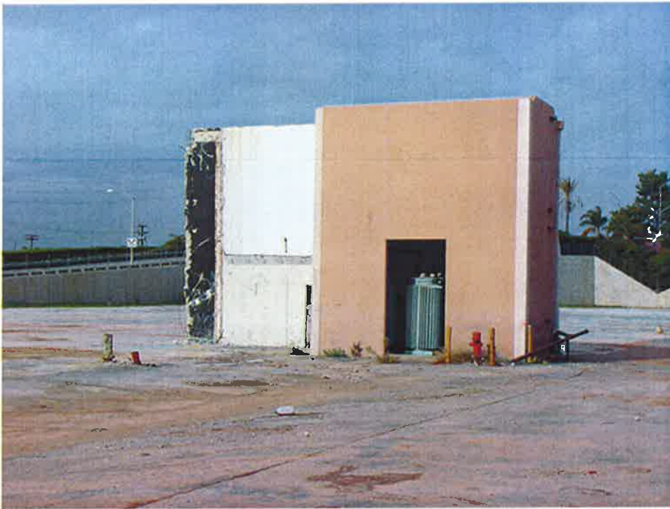
Remaining structure around western substation.
