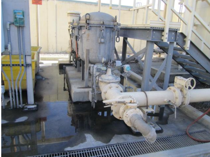
Photo 8. Backwash/recycle equipment
